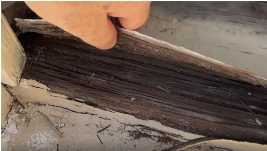
Prior to restoring windowsill and window.
