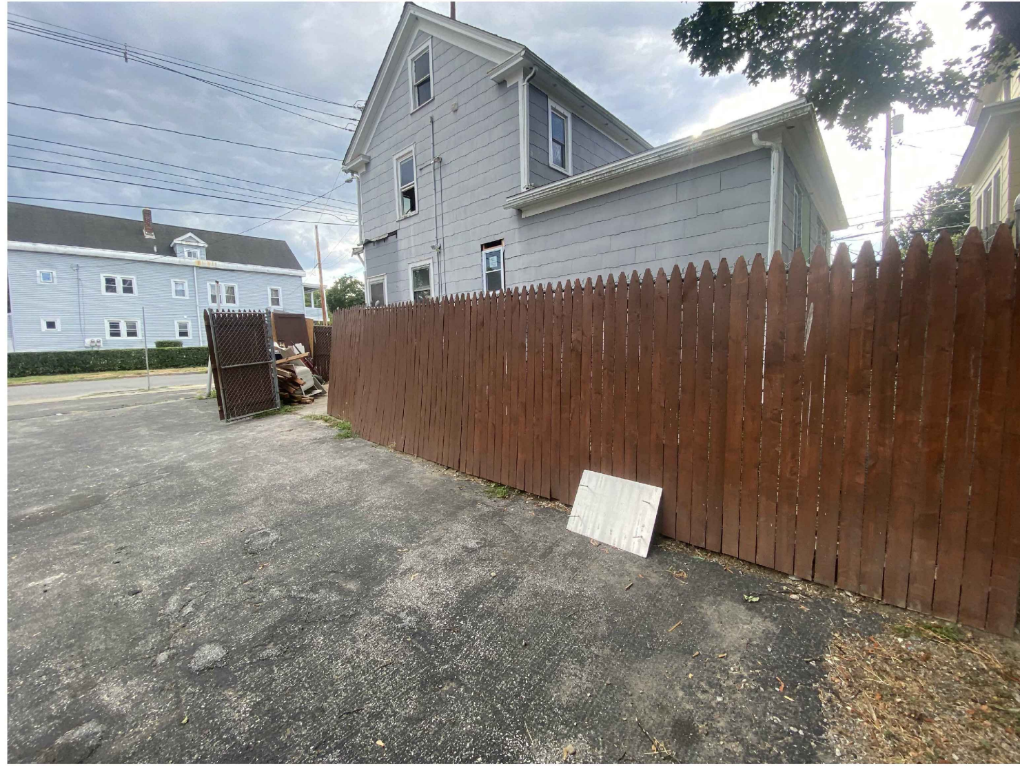
5 67 WORRALL AVE VIEW (rear of building looking south)
