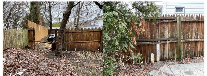
Missing/damaged areas of stockade along western side
