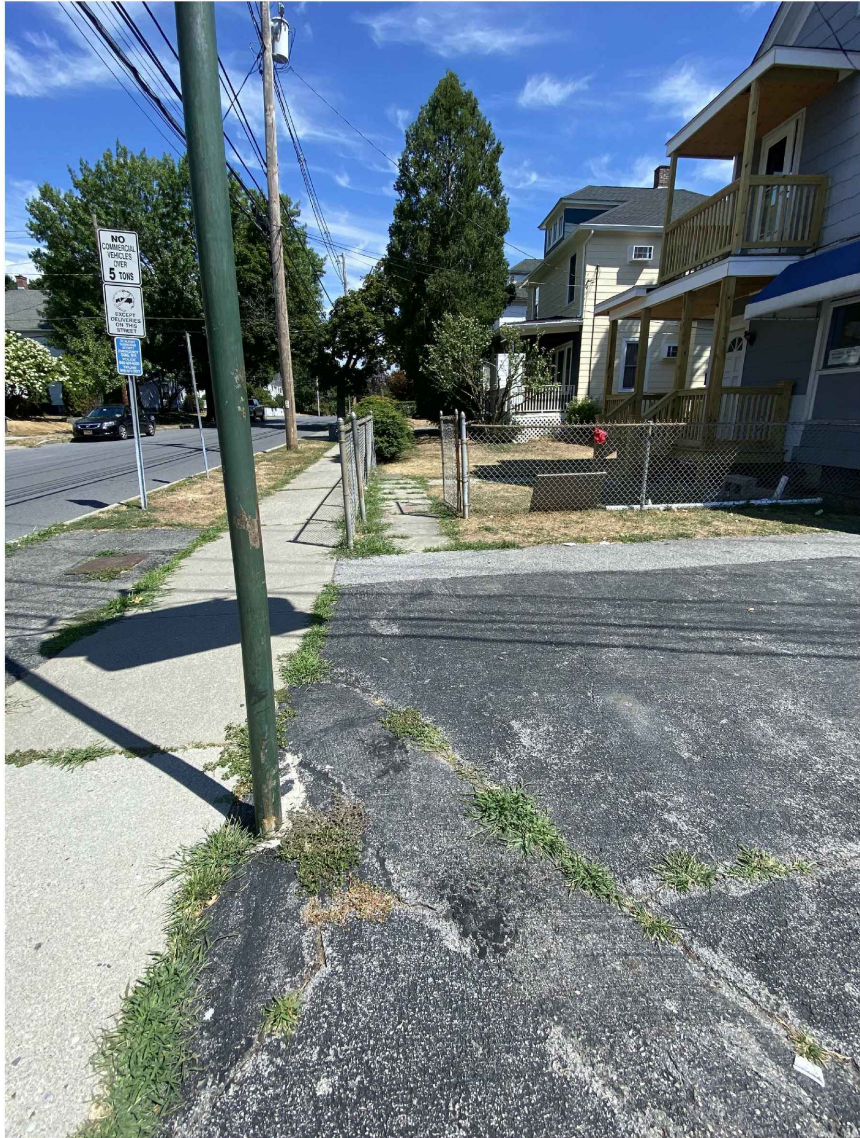
2 67 WORRALL AVE (looking north)
