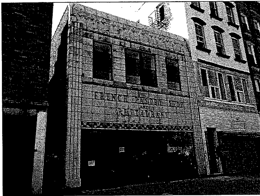
Front (north) facade
