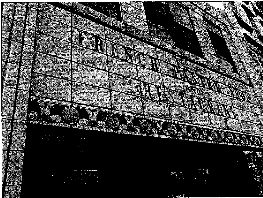
Signage and polychrome terra cotta band over modern storefront
