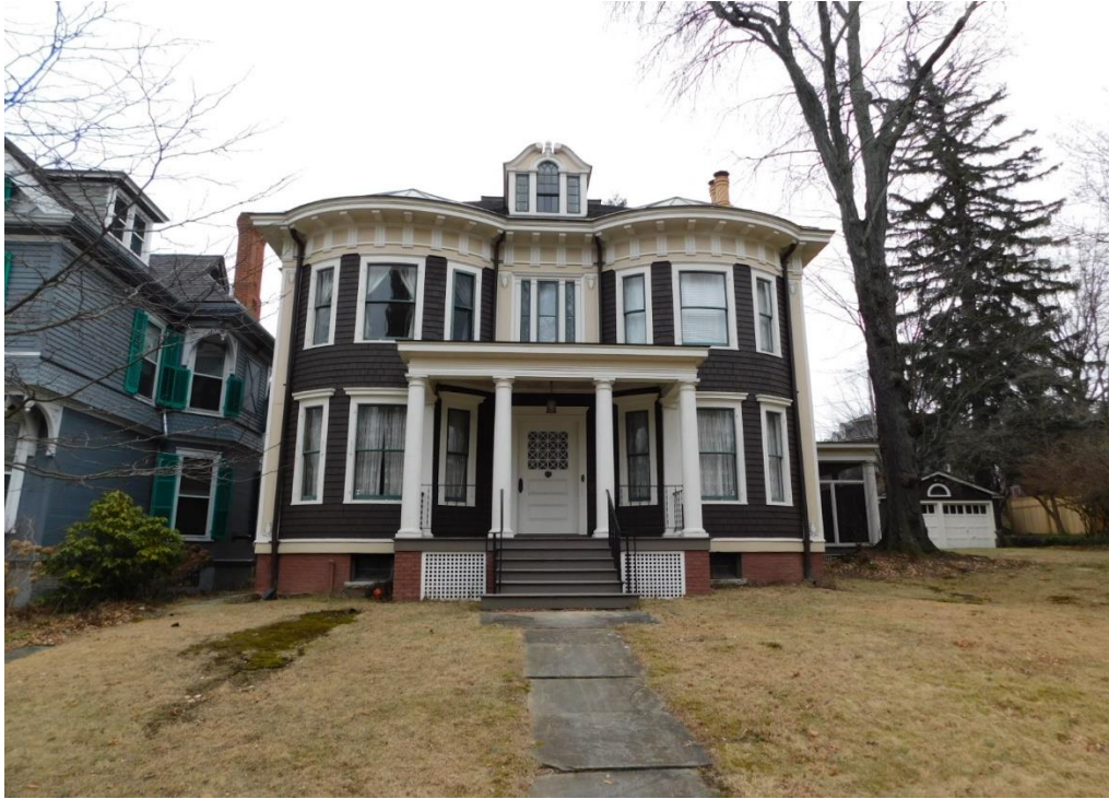
FRONT (WEST) SIDE OF HOUSE
