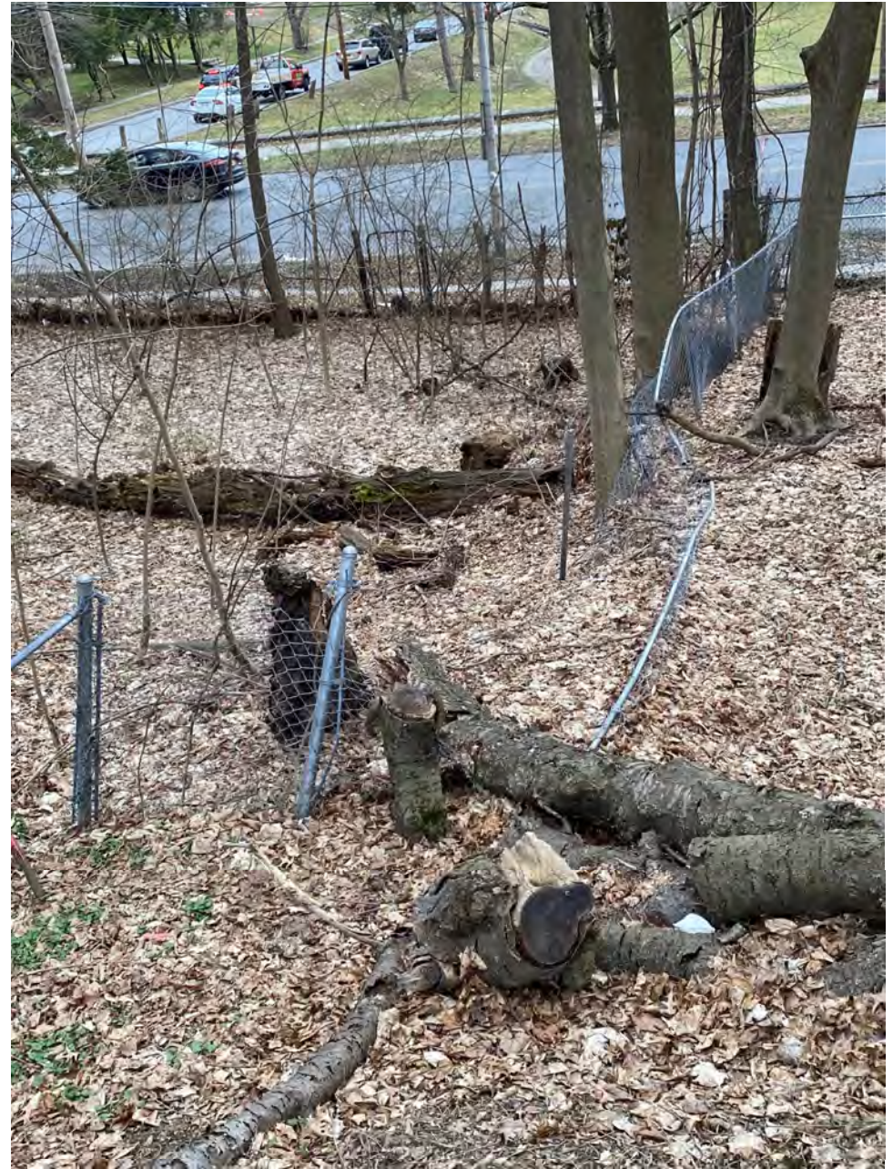
Damaged Fence, South Property Line
