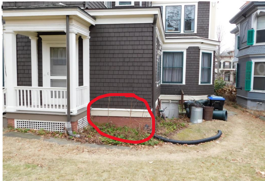
1 LOCATION OF AIR CONDITIONING UNITS - REAR OF HOUSE TO THE RIGHT (NORTH) OF BACK PORCH
