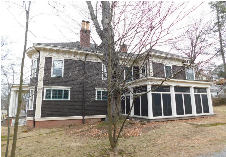
SOUTH SIDE OF HOUSE
