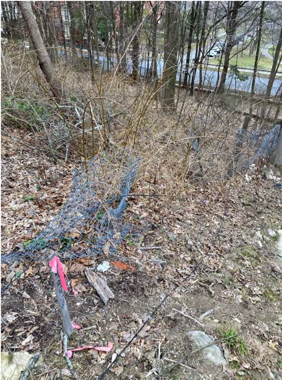
Damaged Fence, South Property Line
