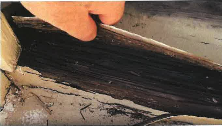
Prior to restoring windowsill and window.
