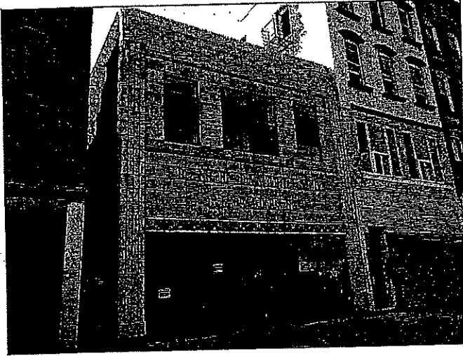
Front (north) facade
