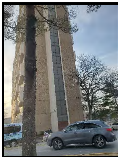
Subject side exterior
