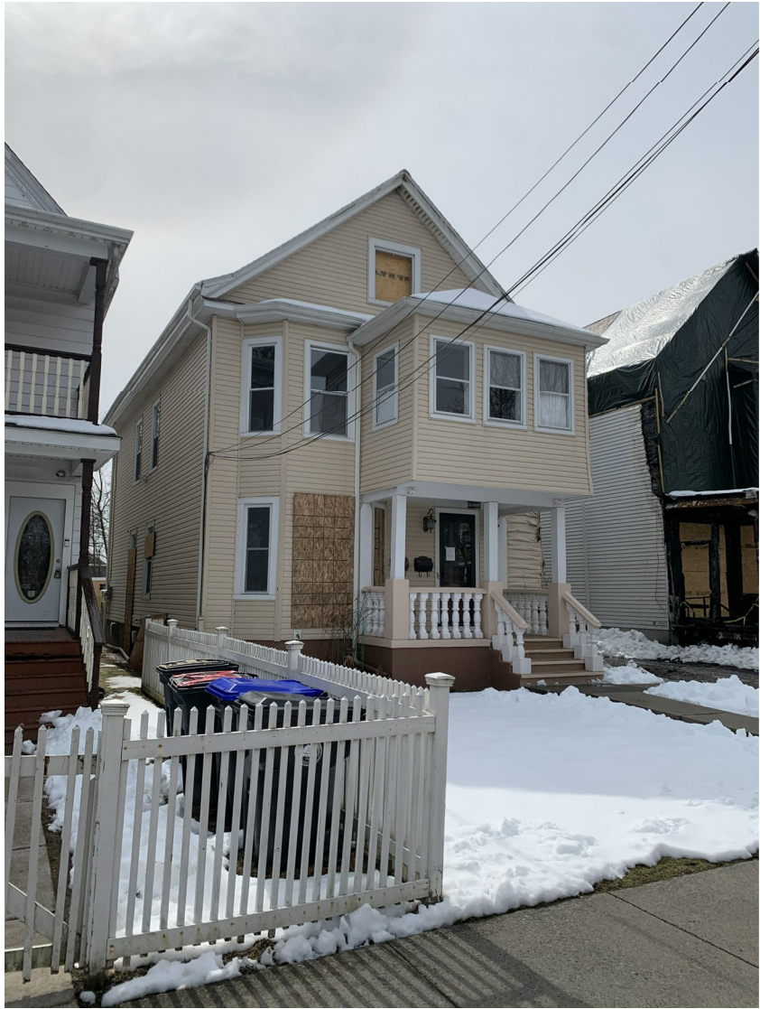
2 Front Facade Photo NTS
