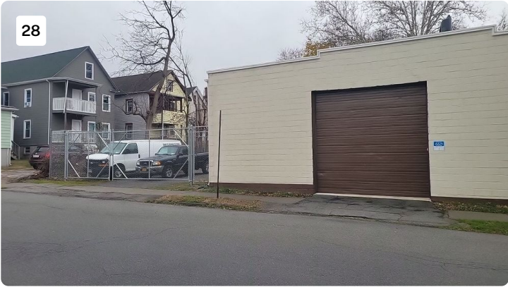
Project: 1 Cottage Street Date: 11/30/2022, 9:20am Creator: Danielle LeClerc
