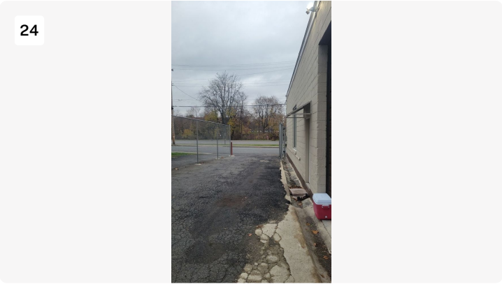
Project: 1 Cottage Street Date: 11/30/2022, 9:18am Creator: Danielle LeClerc
