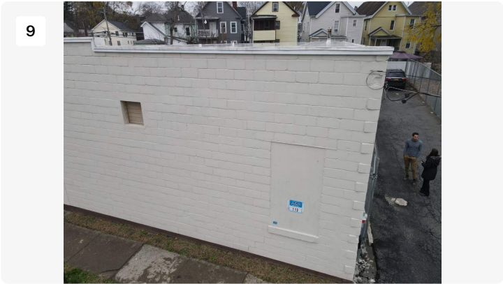
Project: 1 Cottage Street Date: 11/30/2022, 9:13am Creator: Gary Beck
