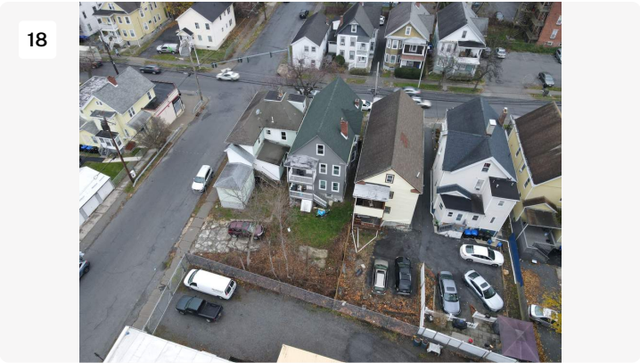
Project: 1 Cottage Street Date: 11/30/2022, 9:15am Creator: Gary Beck
