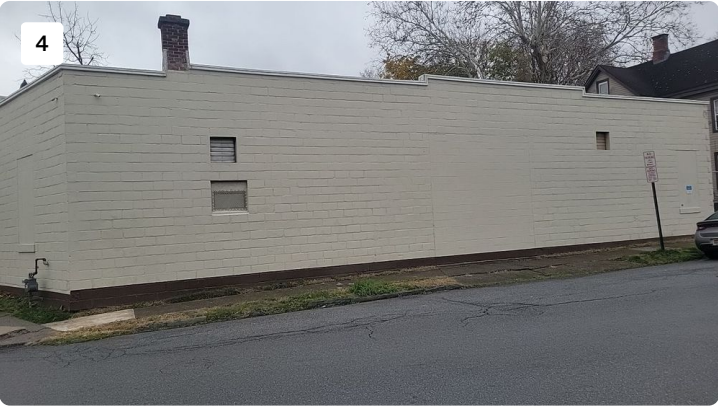
Project: 1 Cottage Street Date: 11/30/2022, 9:12am Creator: Danielle LeClerc
