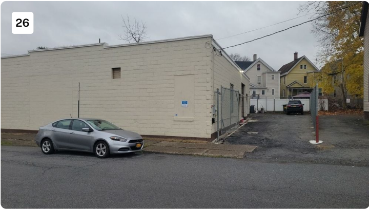
Project: 1 Cottage Street Date: 11/30/2022, 9:19am Creator: Danielle LeClerc
