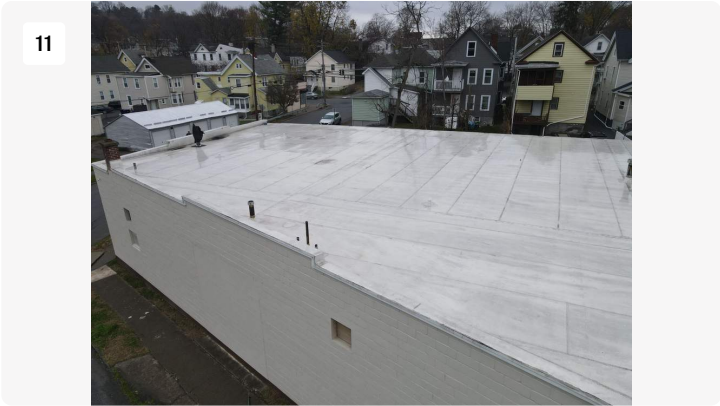
Project: 1 Cottage Street Date: 11/30/2022, 9:14am Creator: Gary Beck
