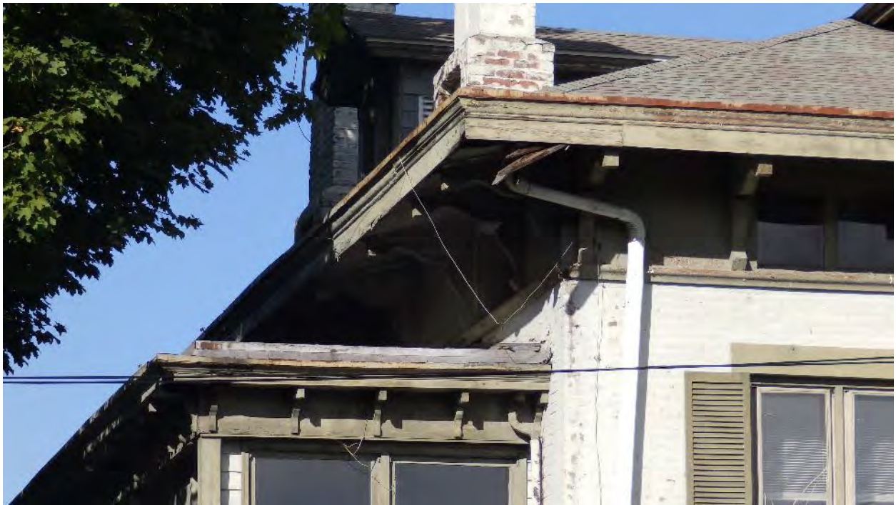
Photo 8: The wide cornice brackets under the eaves have been replaced and designed to match the smaller cornice brackets featured on the porch addition. The eaves have been fitted with aluminum drain spouts. The plywood used in the mid-20th century renovation is rotting away in several locations. View west of the southeast corner of Hill House.
