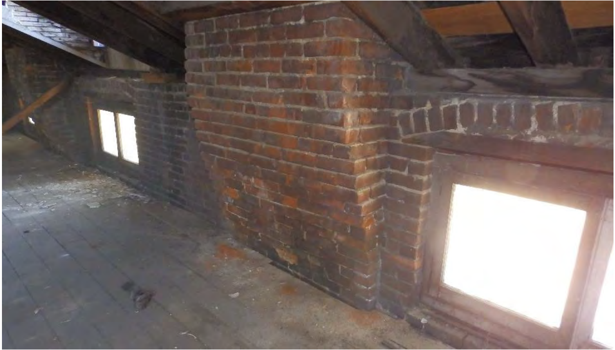
Photo 33: Four chimney can be identified within the attic space. View of the attic windows and chimneys located on the northern elevation.
