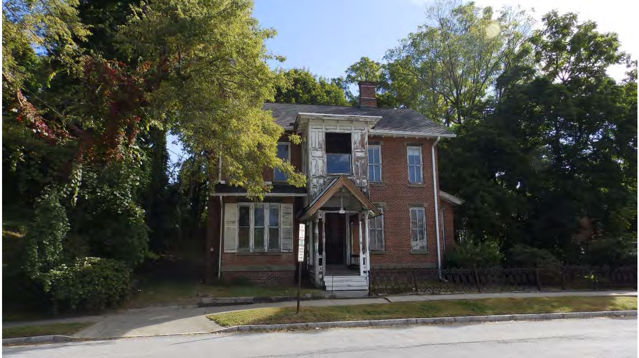
Photo 1: Vacant residential structure located at 18 Davies Place. View to the east. Structure is listed as part of the North Clover-Mill Street District.
