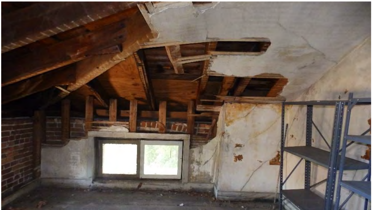
Photo 32: Attic room located on at the southeastern corner of the house. The room shows the original plaster and lathe over brick construction. The chimney is located to the right, on the far wall next to the steel shelves. The window appears to be a mid-20 th century replacement.
