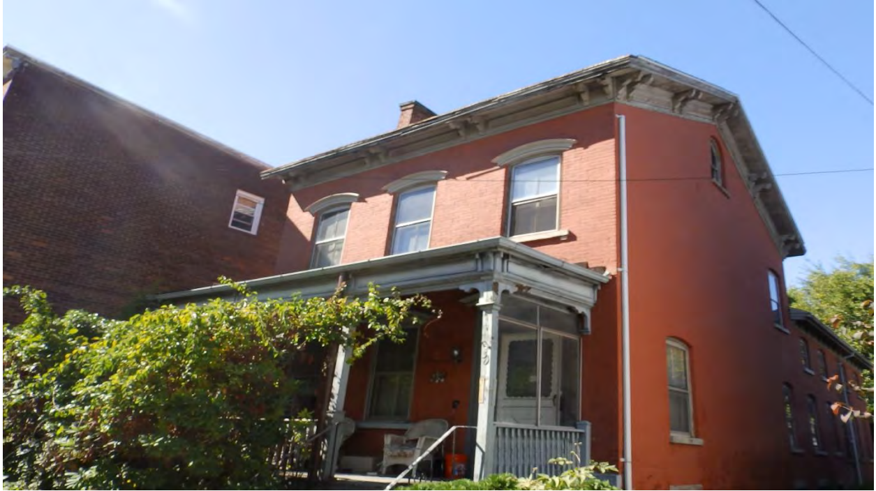
Photo 13: Residential structure located at 30 North Clover Street is included in the North Clover Mill Street Historic District. This building retains many of its 19th century stylistic elements.
