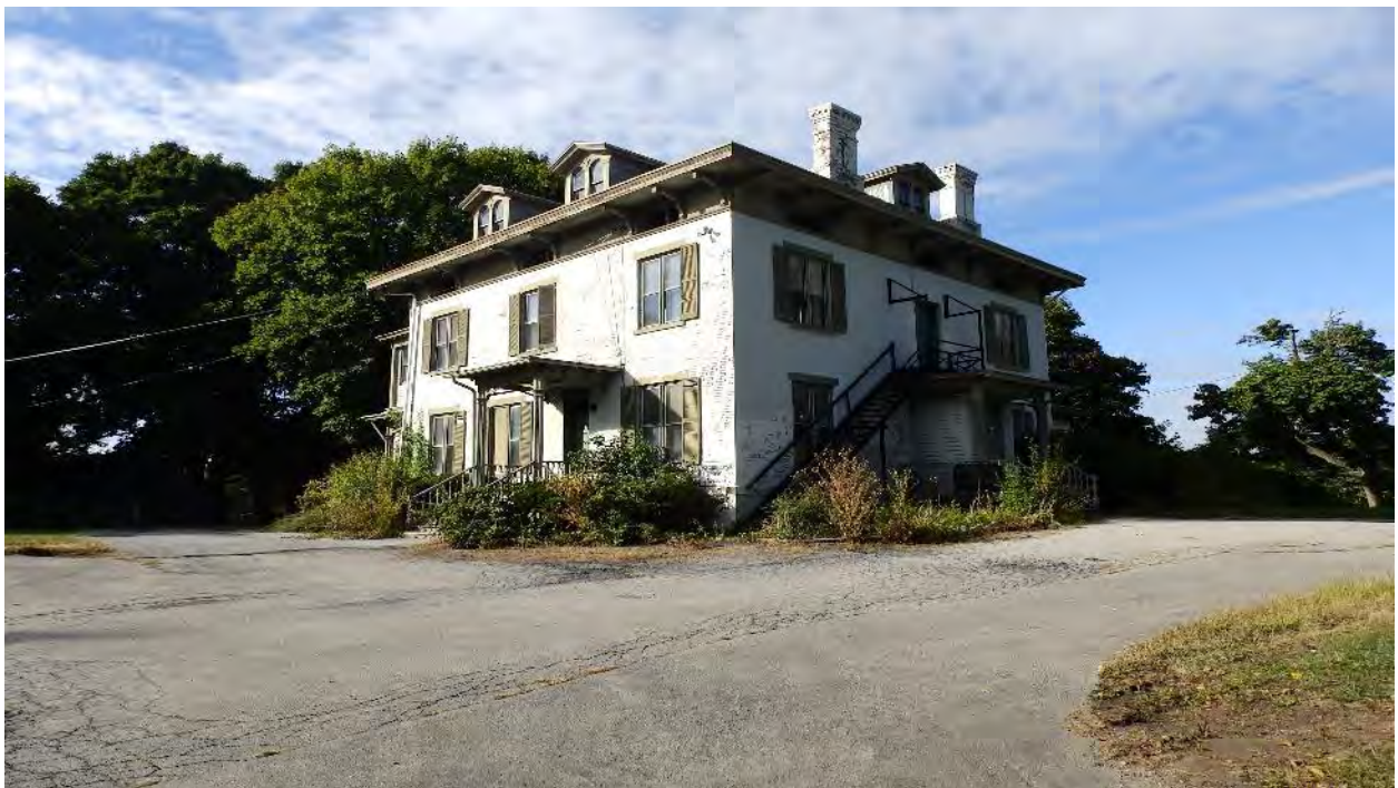
Photo 8: Hill House, an Italianate style structure built in 1859, is located within the central portion of the project area. The house served as the Poughkeepsie Day Nursery School for nearly 100 years. The structure is currently vacant. View to the southwest.
