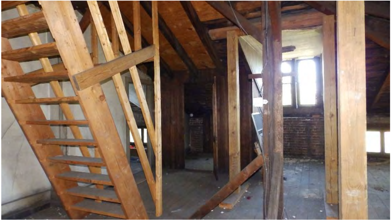
Photo 31: View of the western portion of the third/attic floor. The stairs to the left provide access to the roof.
