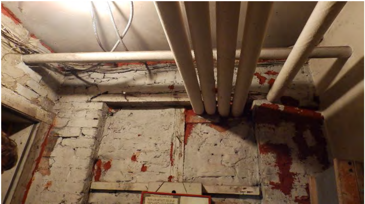
Photo 20: A series of pipes and electrical wires pass through a walled doorway. The area on far side of the wall is identified on the basement floor plan as a void/former stairwell.
