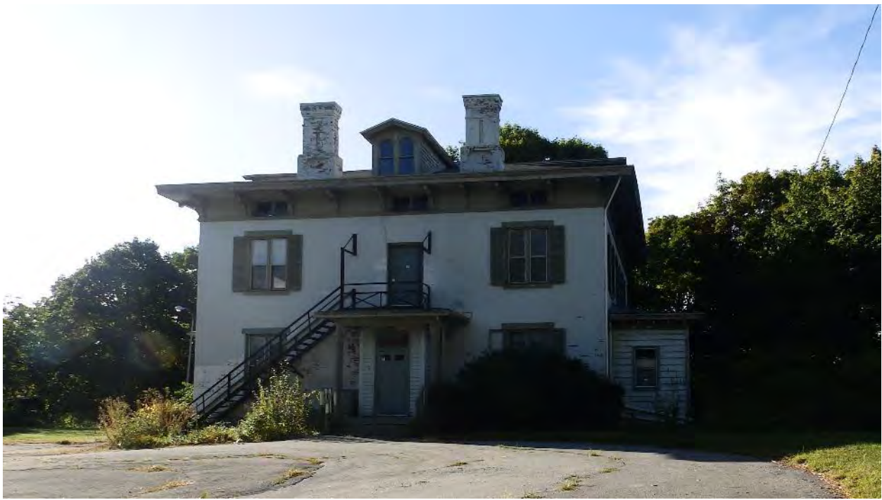
Photo 1: The northern elevation of Hill House. The fire escape and associated doorway were added to the original structure in the mid-20th century. The shutters on the windows, as well as the small porch and wooden entryway also represent 20th century additions to the building. .
