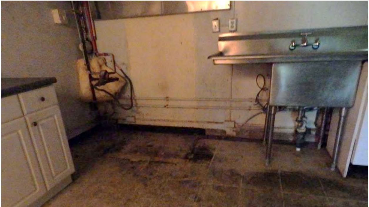
Photo 19: A kitchen is located in southeastern corner of basement area. The materials show extensive upgrades to modernize the room.
