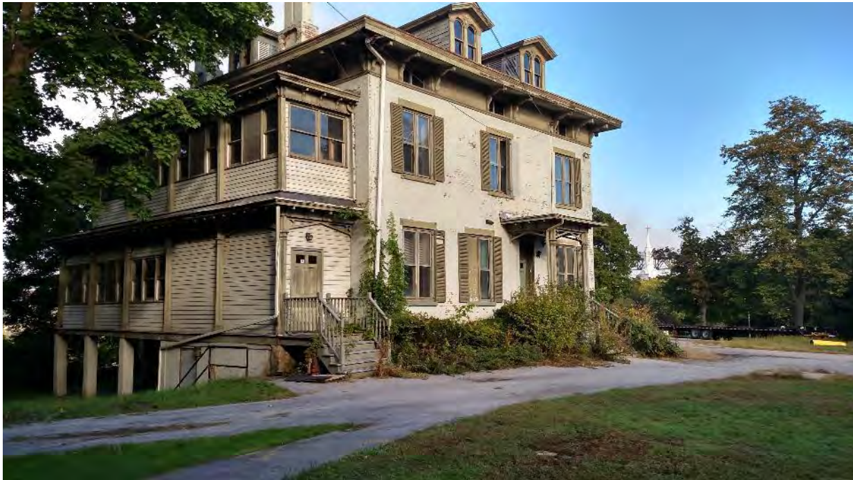
Photo 2: The eastern and southern elevations of Hill House. View to the north.
