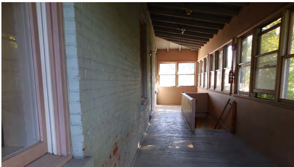
Photo 30: The second story of the veranda/porch. Originally constructed in 1916, this feature was rebuilt after the 1979 fire. The second floor plan identifies the area as room 207. View east of stairs descending to entrance on the first floor.
