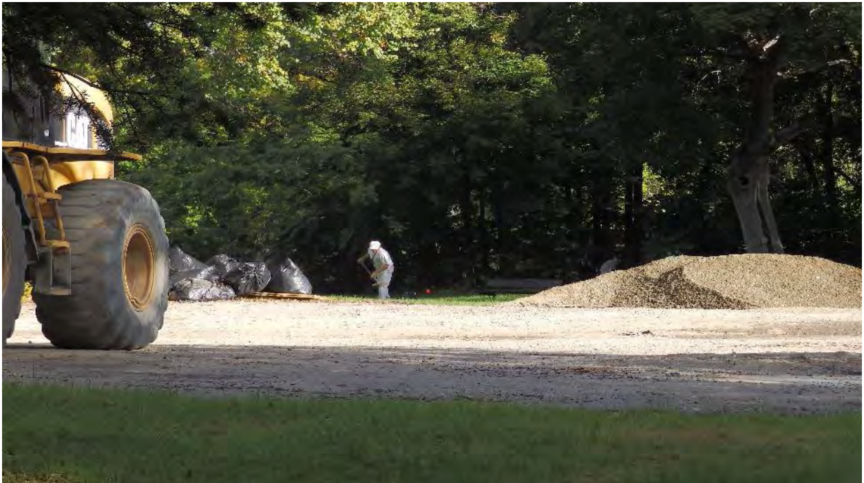
Photo 14: Field Technicians completing shovel tests along TR 6. The site is currently being used for equipment and supply storage for the City of Poughkeepsie's improvement of North Clover Street. View to the east.
