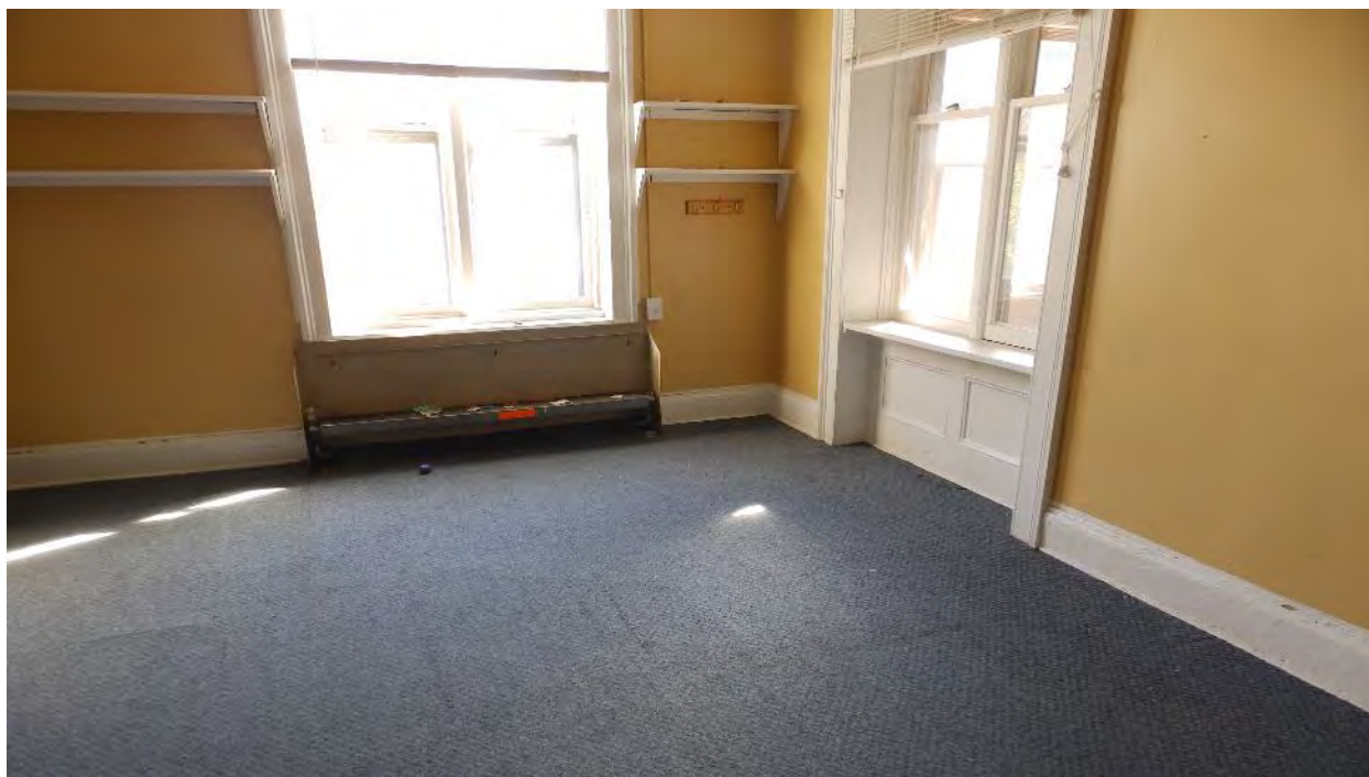
Photo 29: This room is identified on the Second Floor Plan as 209. As with the other interior rooms, the floor has been carpeted and the original walls have been replaced with sheetrock.
