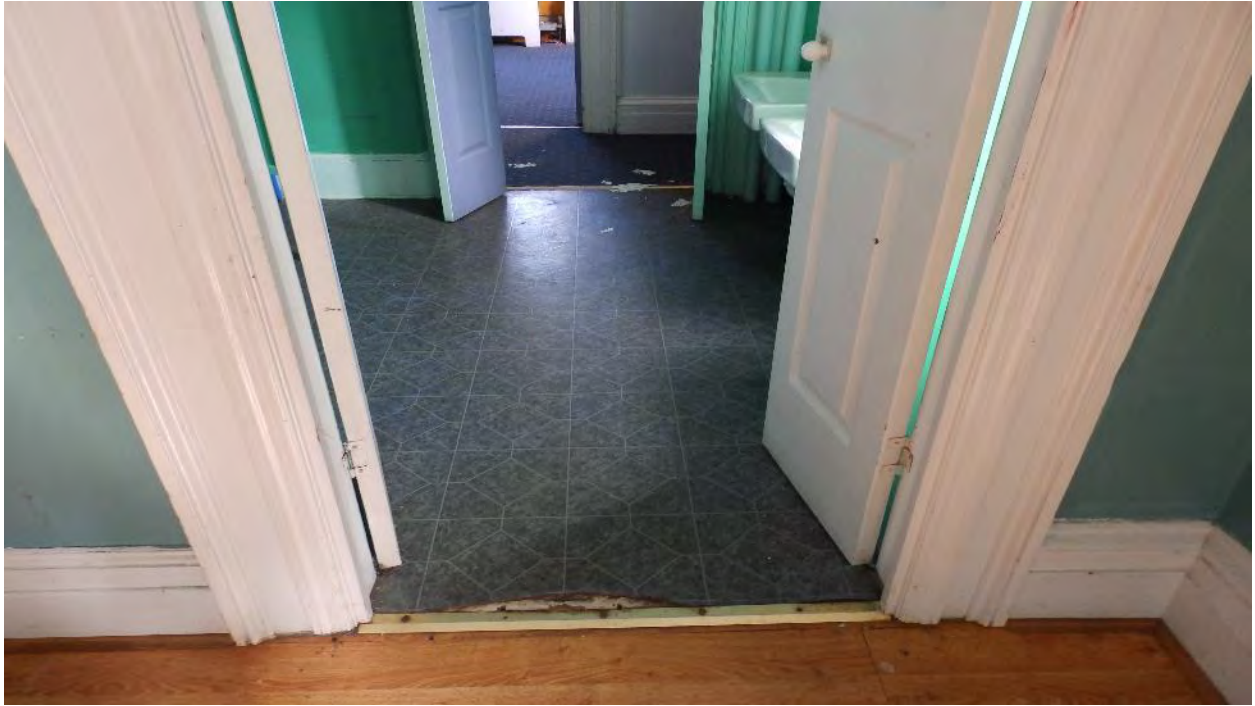
Photo 23: This room is identified on First Floor Plan as 105, and is the first floor bathroom. Changes along the floor trim suggest the linoleum is laid over plywood.
