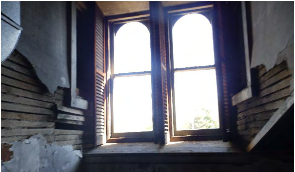
Photo 32: View east from the arched window in eastern attic elevation. The arched side windows are present, but have been covered. Windows are shuttered from the inside, and appear original.
