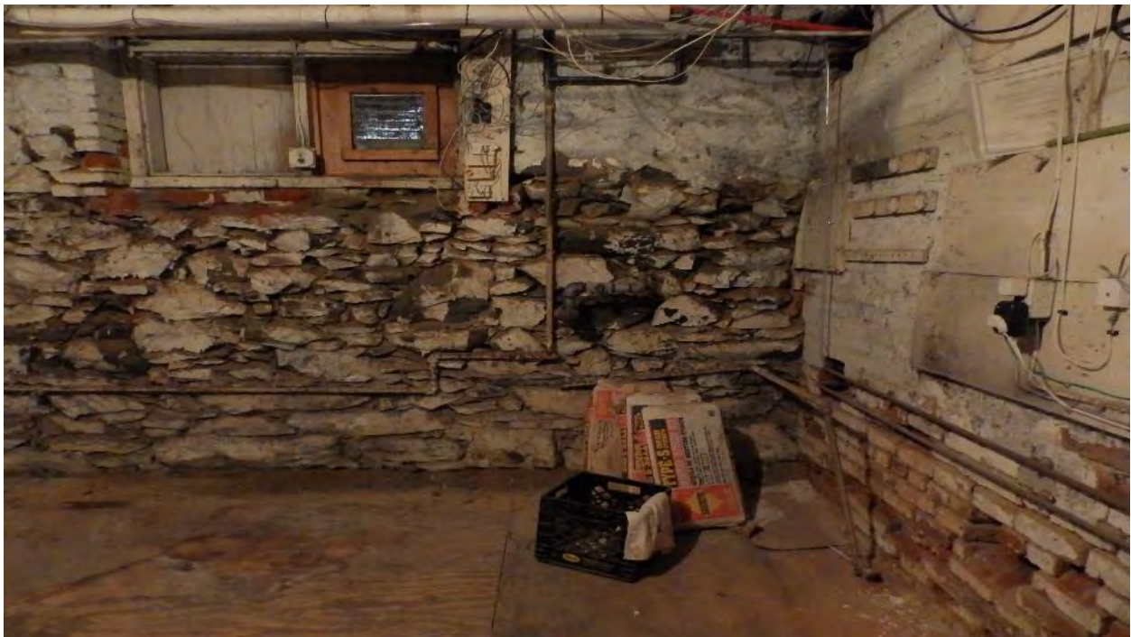
Photo 16: The room identified on floor plan as Storage 06, is a below grade room constructed of brick and fieldstone. Framing around the window on the far wall appears to be original. View to the east.
