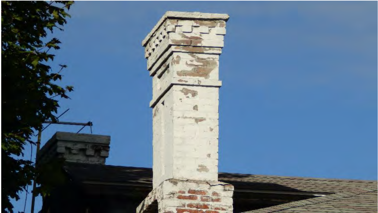
Photo 7: Four ornately decorated brick chimneys are located at each of the four corners of the hipped roof. The chimneys feature a dentil pattern at the top edge. View to the west of the chimneys at southern portion of the house.
