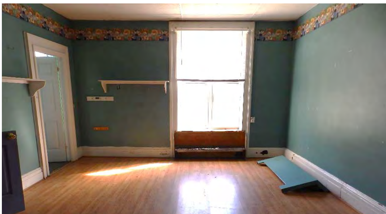
Photo 22: This room is identified on the First Floor Plan as 107. Patching along the floor trim suggests that a fireplace was once located in the area where heating register cover is laying on the floor. View to the east.
