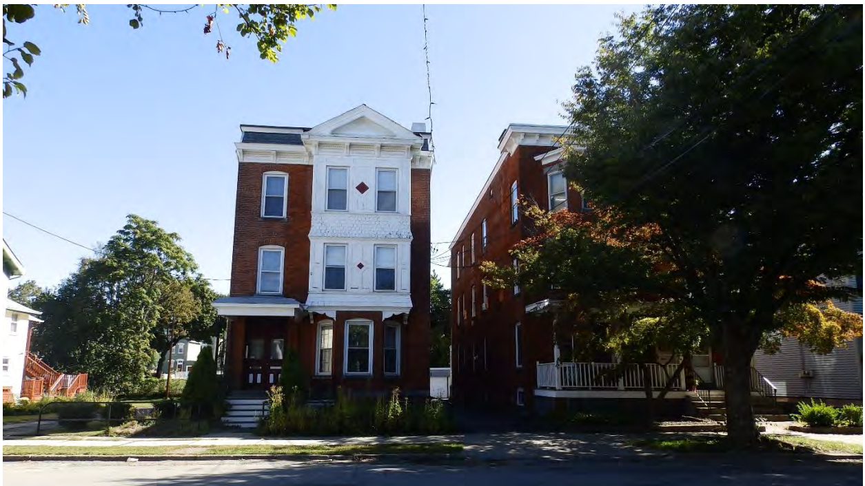
Photo 10: Residential building at 17 North Clover Street. View to the east.
