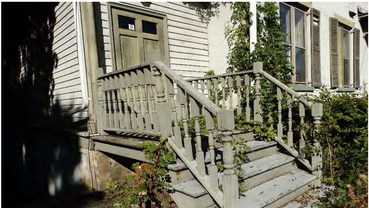
Photo 9: The enclosure of the original veranda included the construction of a new entryway. This area was damaged by a fire in 1974 and was subsequently rebuilt. View of the first level entry to the porch on the south elevation.
