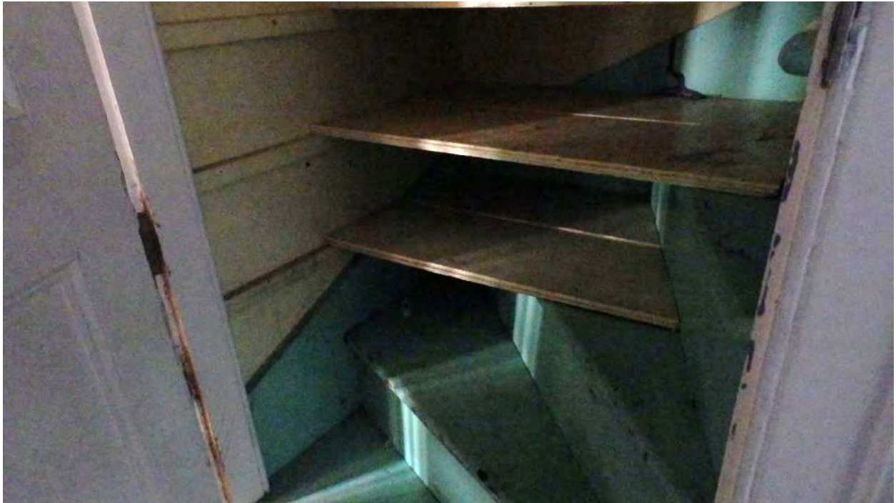
Photo 25: The original servant's stairwell has been converted into a storage closet. Identified on the First Floor plan as adjacent to Room 106, which is a small hallway.
