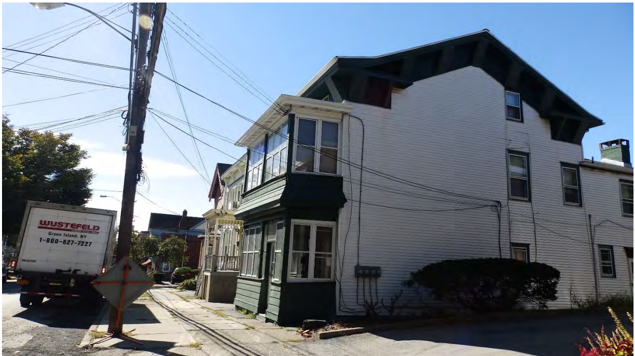
Photo 12: Residential Structures located at 12-16 North Clover Street are included in the North Clover Mill Street Historic District. Although many original historic elements remain these structures have been upgraded with modern materials.
