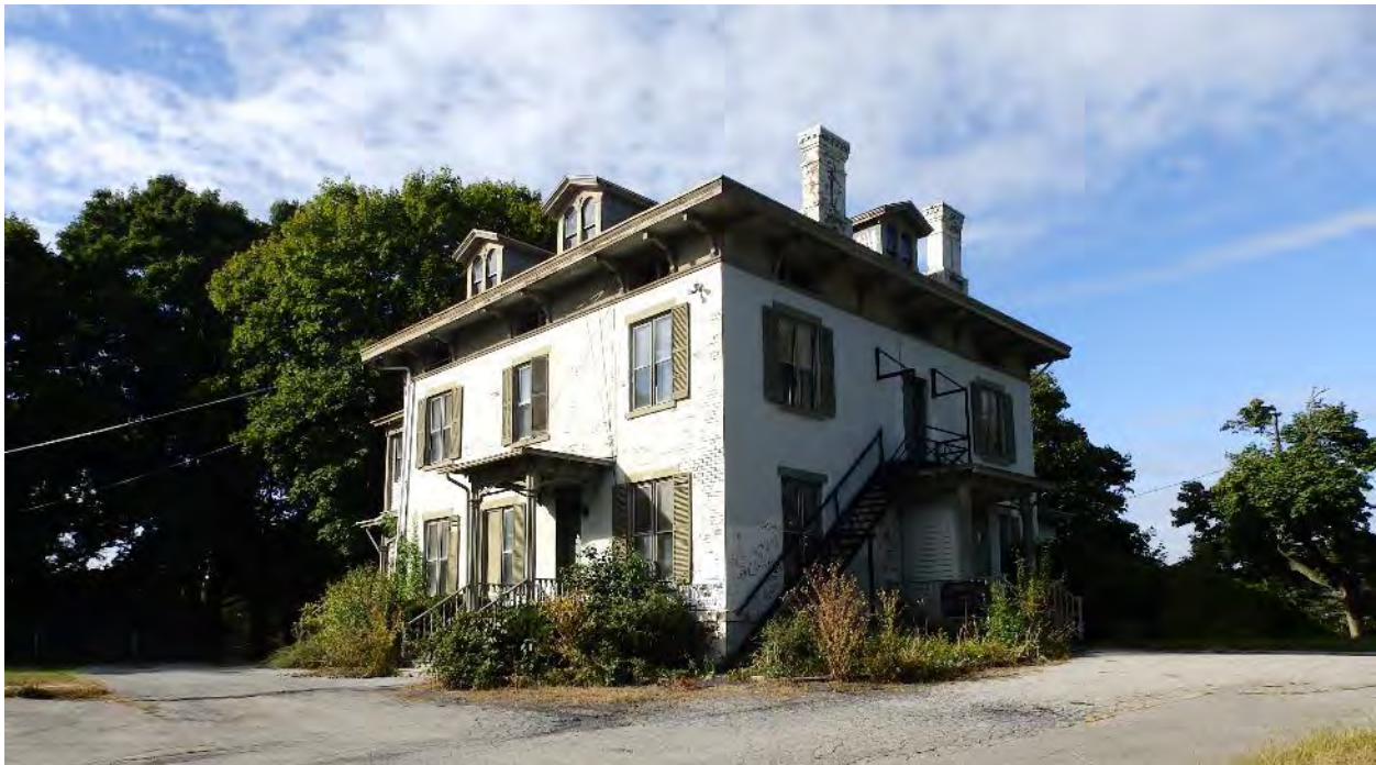
Photo 14: 2015 Photograph of Hill House showing the eastern and northern elevations. View to the southwest.
