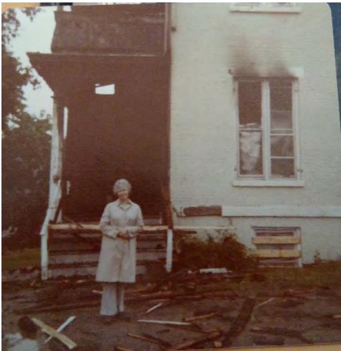
Photo 9: View of the southeastern corner of Hill House after the fire in May 1979. (Source: Poughkeepsie Day Nursery Files: Adriance Memorial Library).
