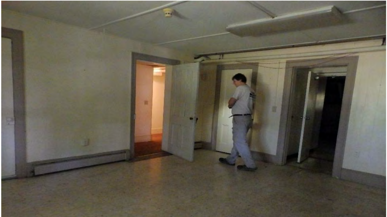
Photo 17: Room identified as Storage 02. View looking toward stairway seen in Photo 15. This room features sheetrock walls, baseboard heating and linoleum flooring. The drop ceiling hides original floor supports. The doorways between the rooms feature modern trim material.
