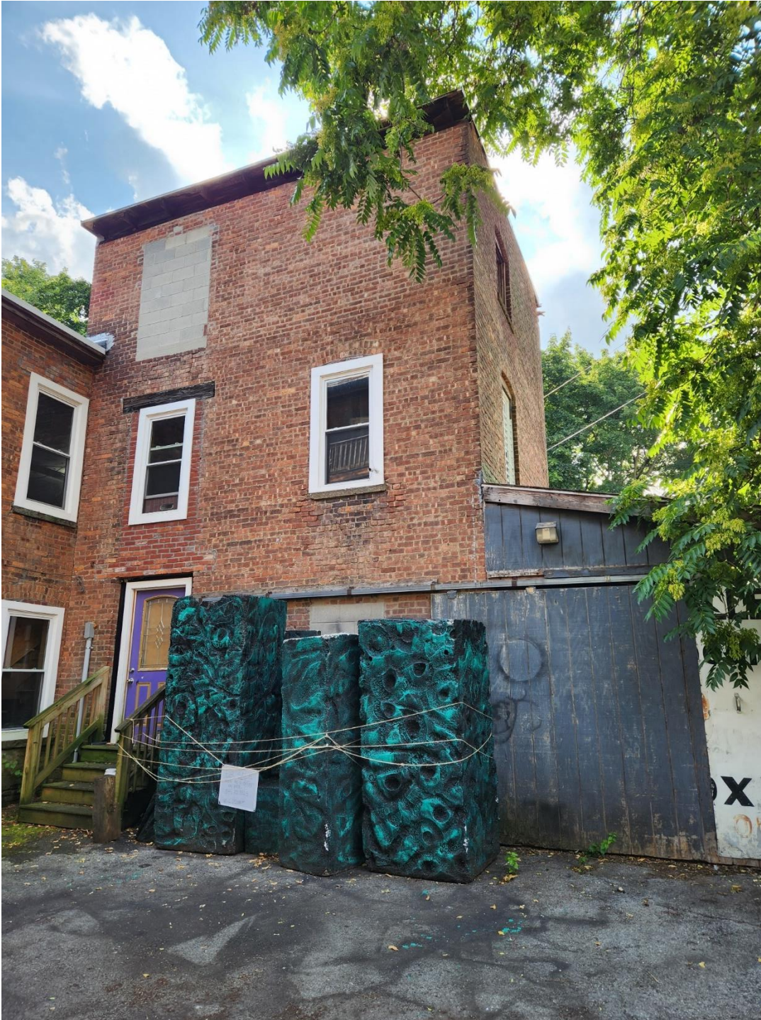
View of rear accessory structure (“carriage house”) from internal courtyard. Third level no longer accessible.
