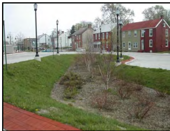
Figure 36: Example of a Bioretention Facility Along Roadway
