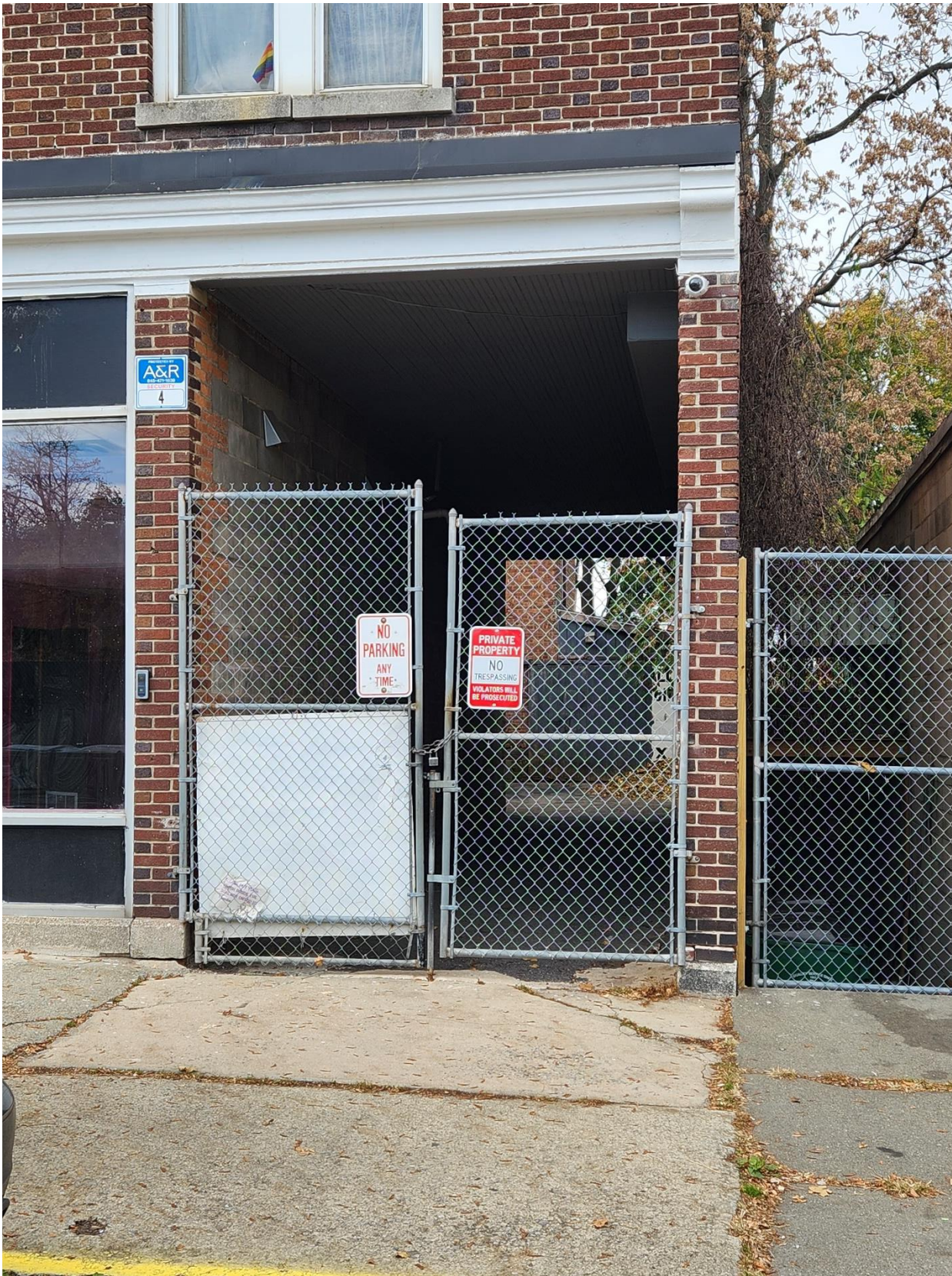
Close up of accessway from sidewalk, leads to internal courtyard and rear accessory building.
