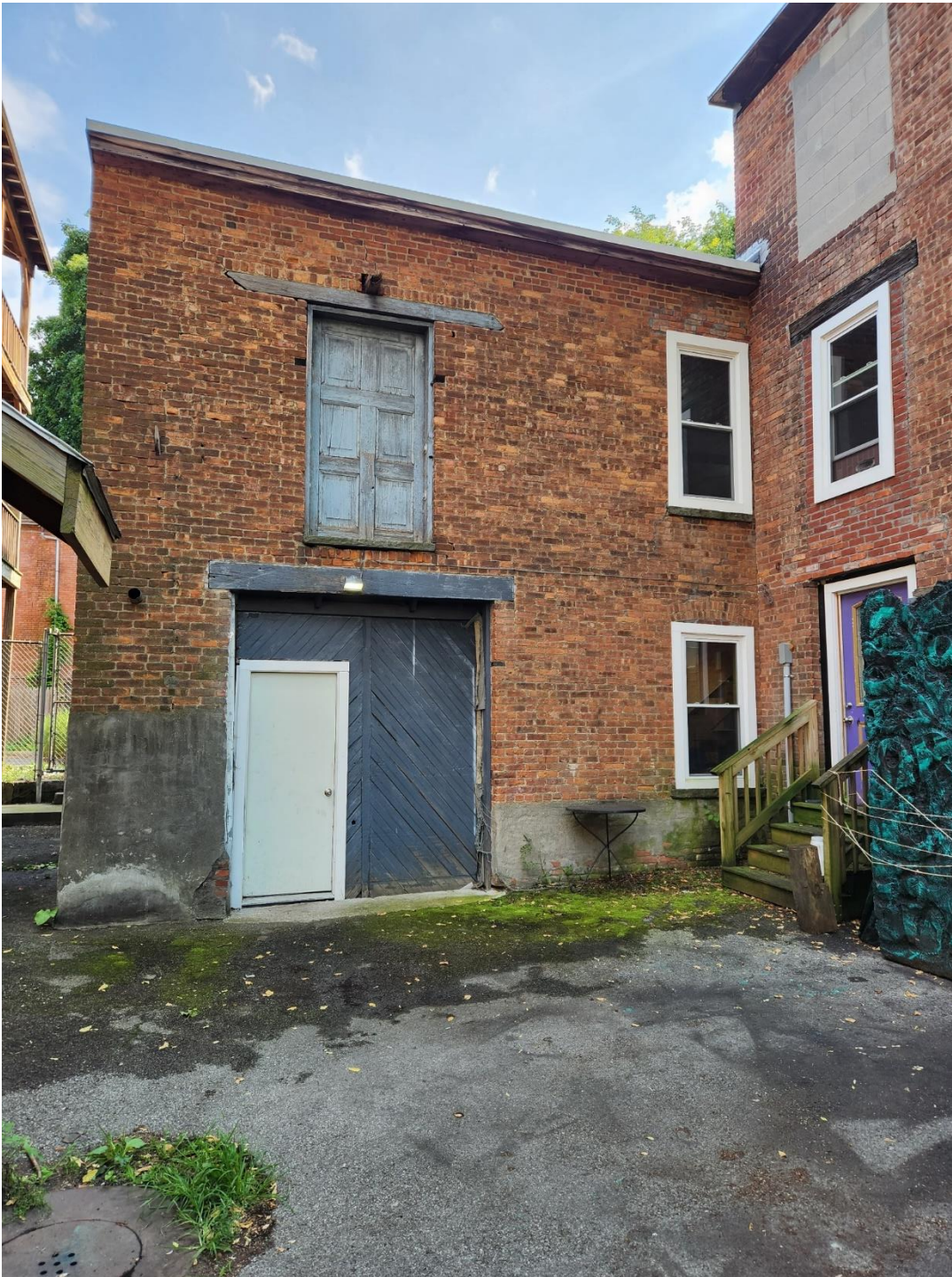
View of rear accessory structure ("carriage house") from internal courtyard
