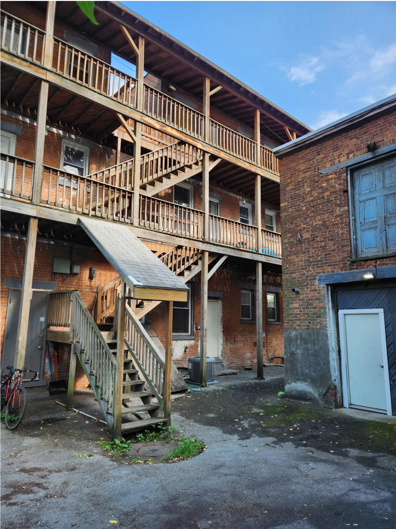
Rear of primary structure from internal courtyard / rear accessory building
