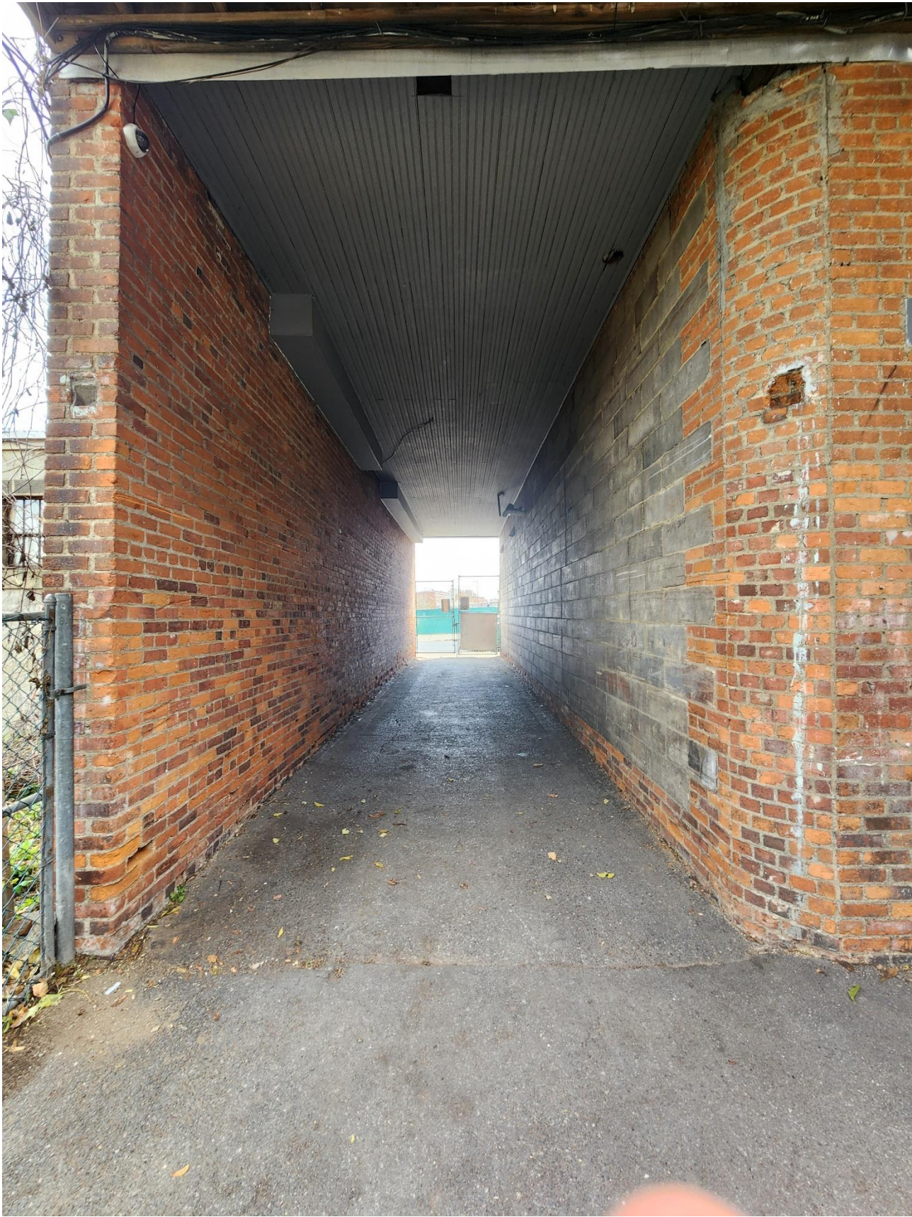
Accessway looking from internal courtyard out towards sidewalk
