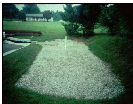
Figure 39: Infiltration Trench (Source: MA EOE, 2005)
