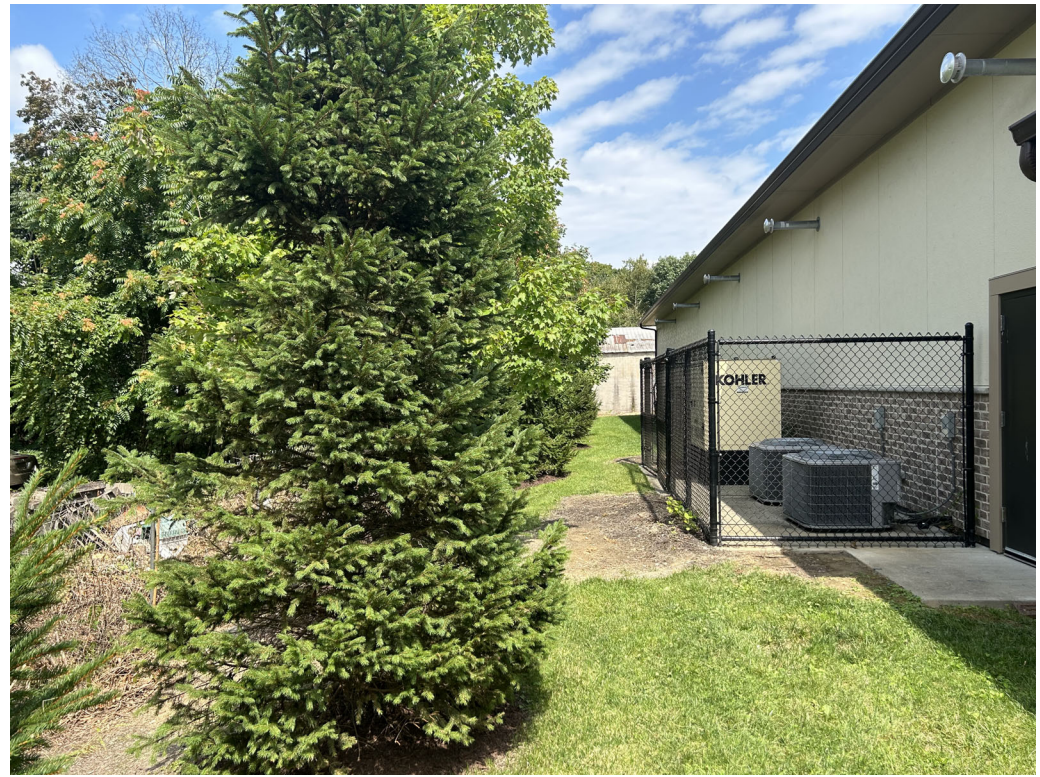
VIEW SOUTH FROM BEHIND THE BUILDING
