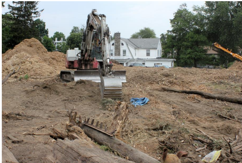
PHOTO 1. Excavating test pit TP4. All photos were taken on June 14, 2023.
