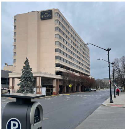
Looking North on Civic Center Plaza
