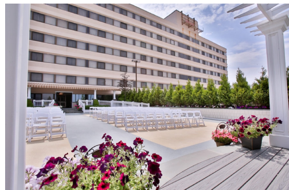
West Elevation from parking ramp
