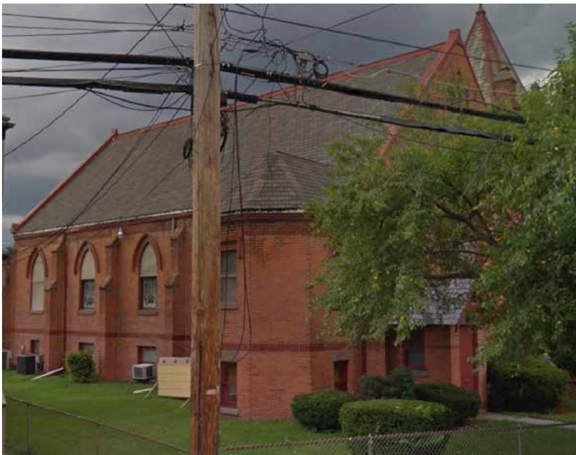
south (side) facade
