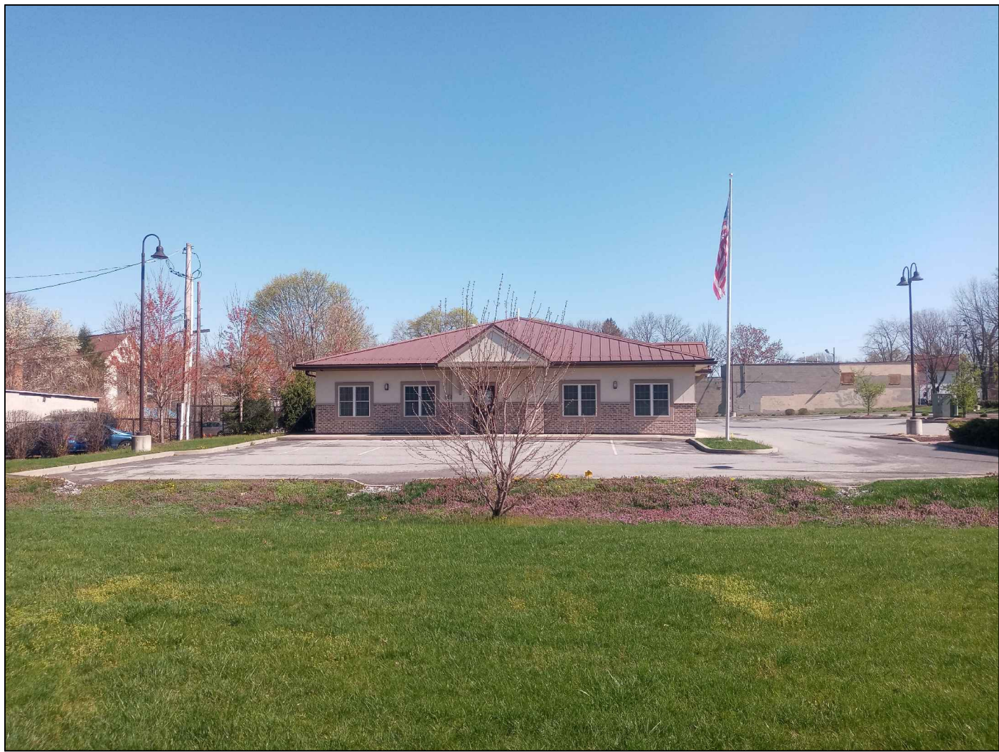
BUILDING NORTH VIEW
