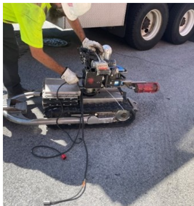
Figure 2: RedZone Robotic LIDAR Scan
