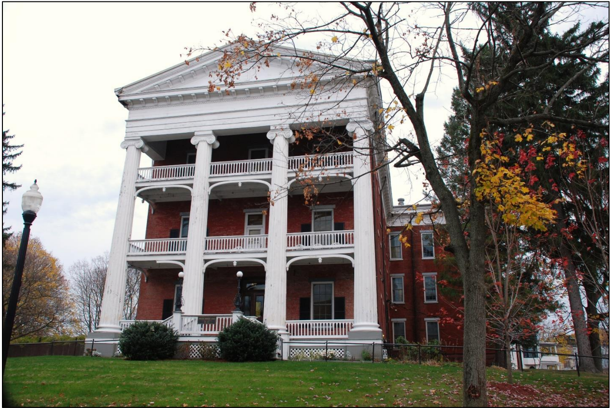
Front West Facade
