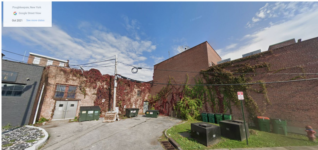
Figure 3: Rear of 306 Main Street and side of 316 Main Street (from Hurlihe St)
