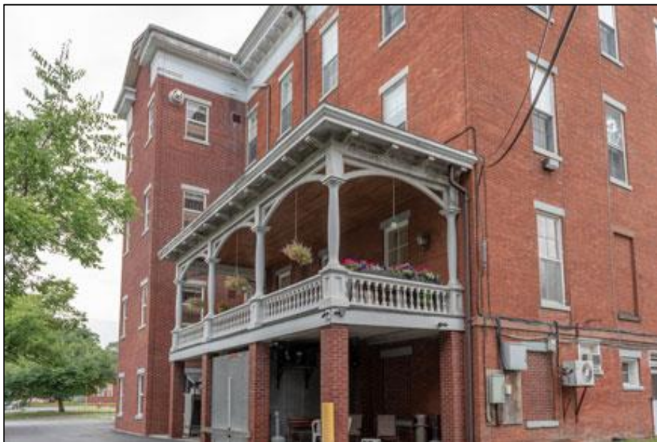
Rear East Facade
