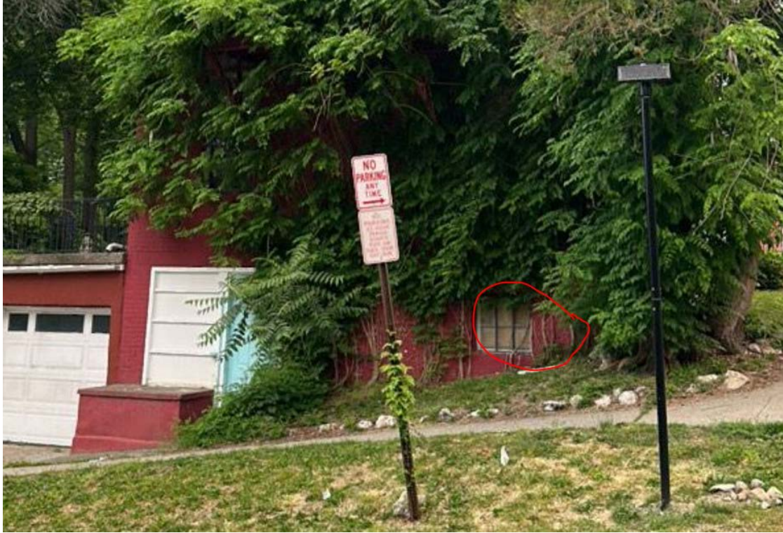
30 Garfield Place Original Basement window
