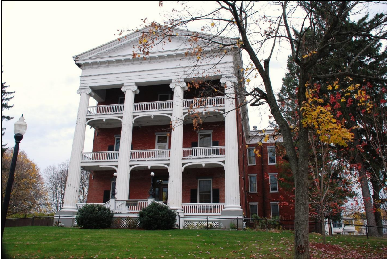
Front West Facade
