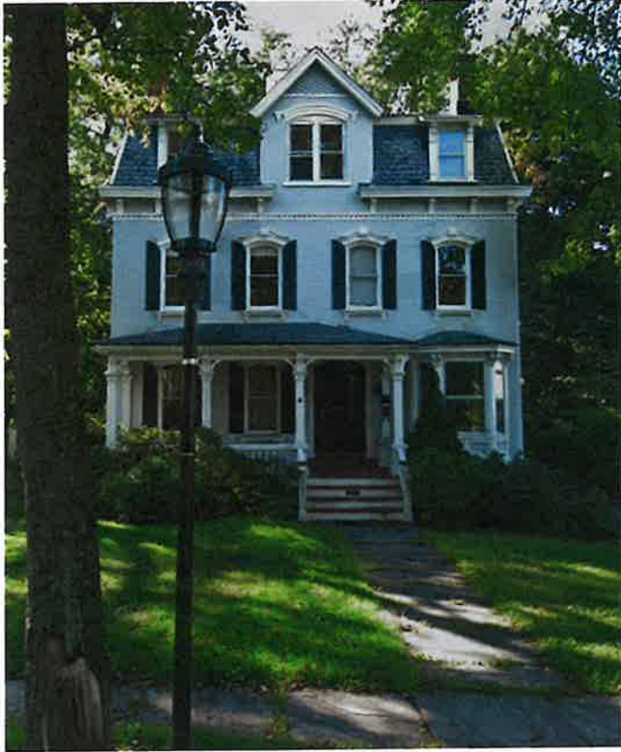
8 Garfield Place, one of the few Spross buildings surviving
