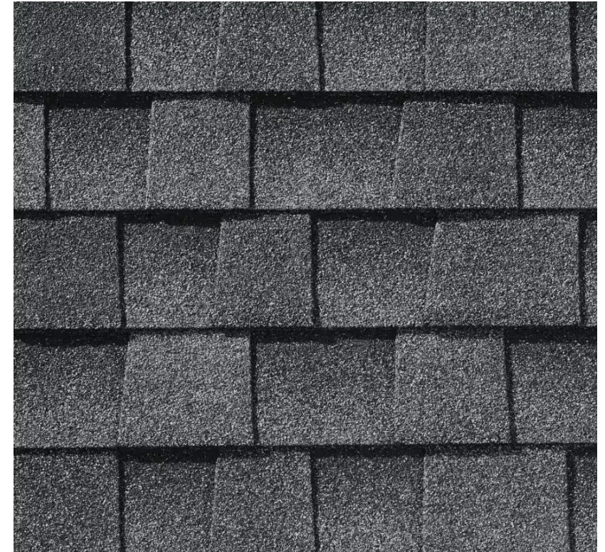
Slate Gray Asphalt Roof Front Porch.
