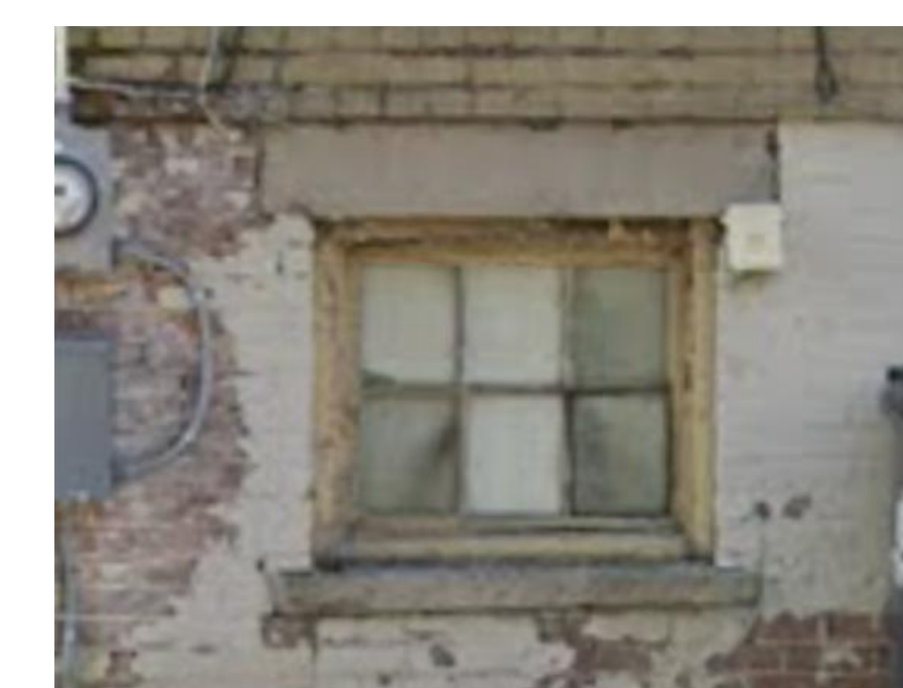
EXISTING BASEMENT WINDOW
