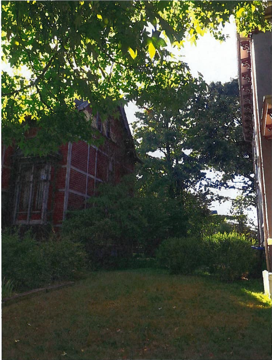
Sidewalk view, 130 Academy north wall .
