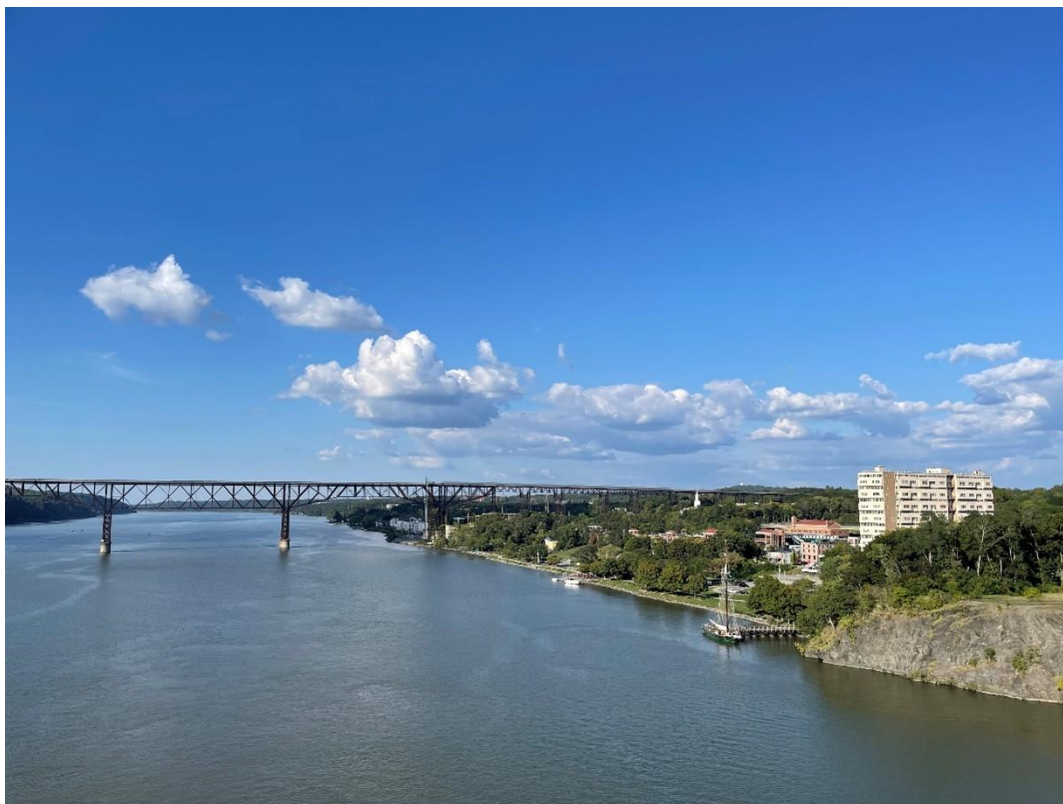
Image 4: View from the Mid-Hudson Bridge looking North toward 141 North Water Street.
