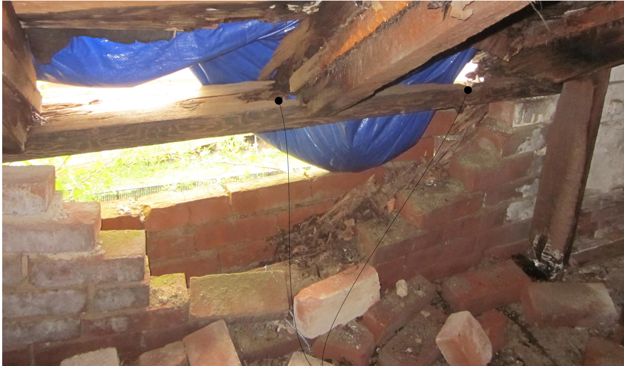
3 INTERIOR VIEW - SOUTH FACADE TOP PLATE N.T.S.
