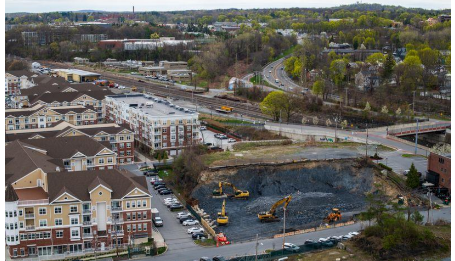
Figure 2: Existing site conditions and view of the bluff 141 N Water Street sits upon.
