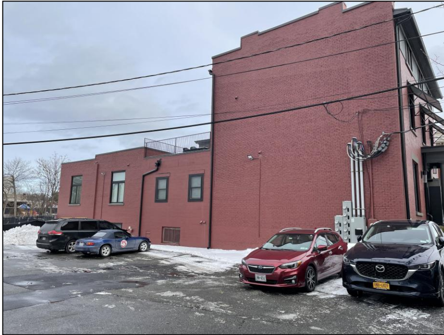
Existing parking at 49 Civic Center Plaza, looking east to 267 Mill Street.
