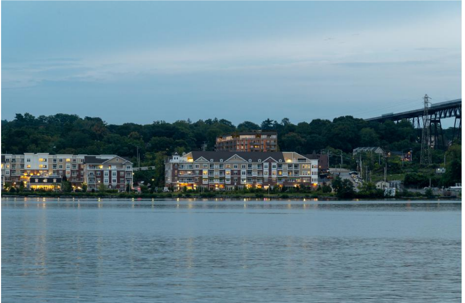
Figure 8: Important waterfront viewshed noting that the elevator penthouse is not visible from this view.
