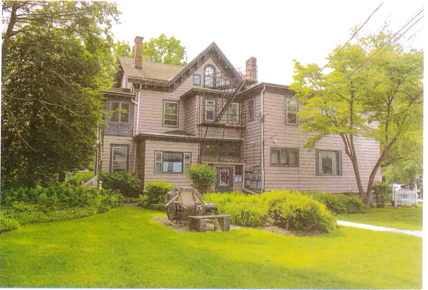
PREVIOUSLY INSTALLED PATIO
