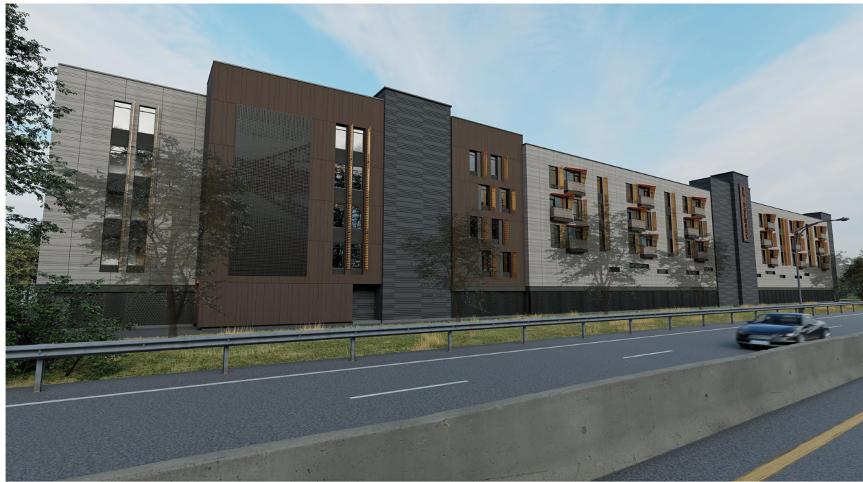
Parking Screening BOK Modern Panels Pattern: Custom or Equal Material: Powder Coated Aluminum Color: BM French Beret 1610
