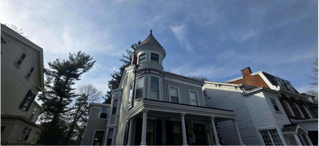
South East side of home
