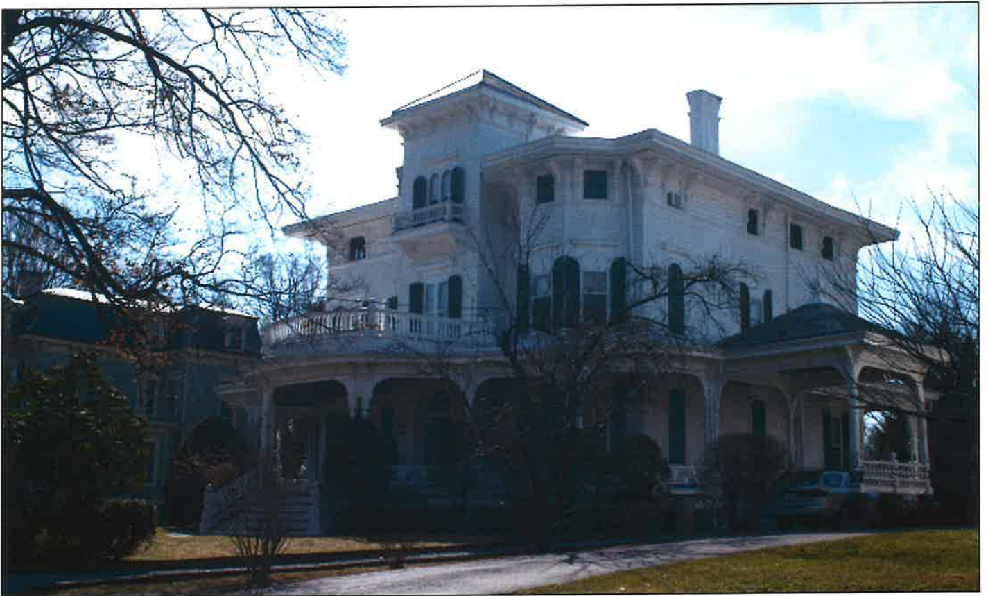
East and North facades
