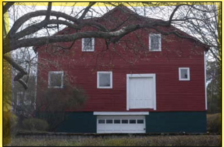
Carriage Barn at 85 S. Hamilton, Carroll St. (west) facade; this barn replaced an older stable on the same site
