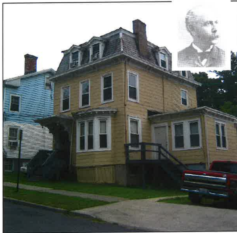
Poughkeepsie Architect Arnout Cannon (inset); and his home at 144 Franklin Street as it looks today
