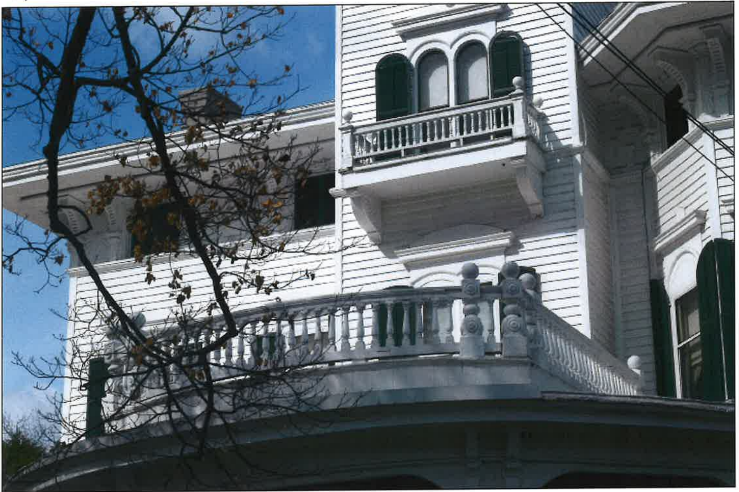
Second and third floor balustrades, cornice brackets, 3rd floor window frieze - on front (east) facade
