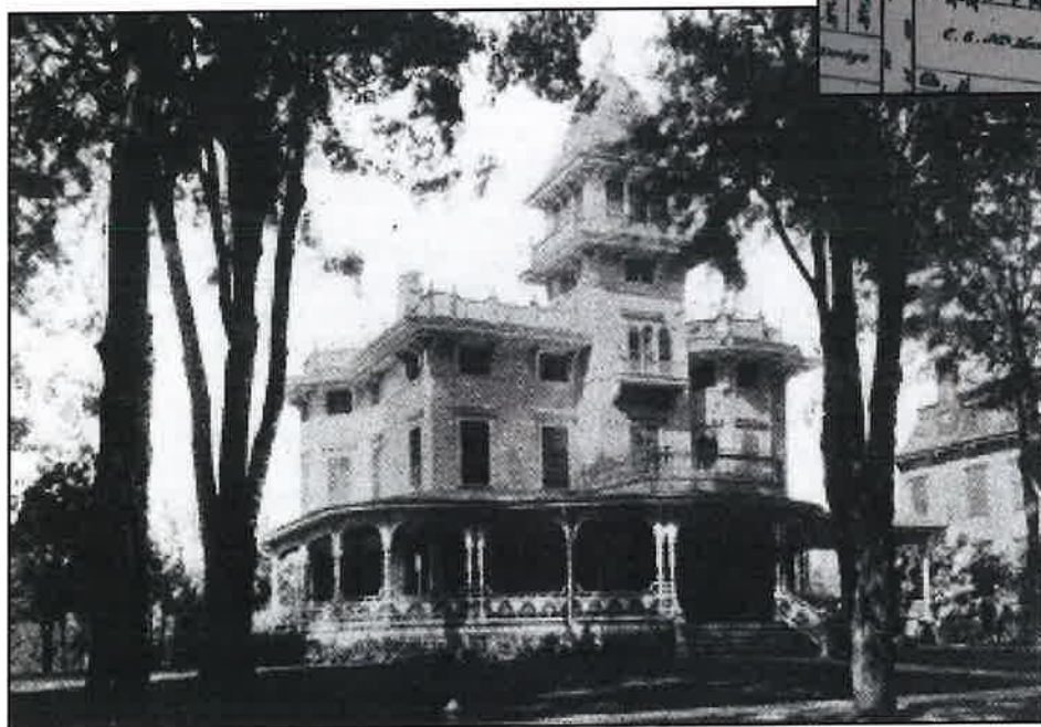
c. 1905 photo of 85 S. Hamilton showing earlier tower design and rooftop balustrade
