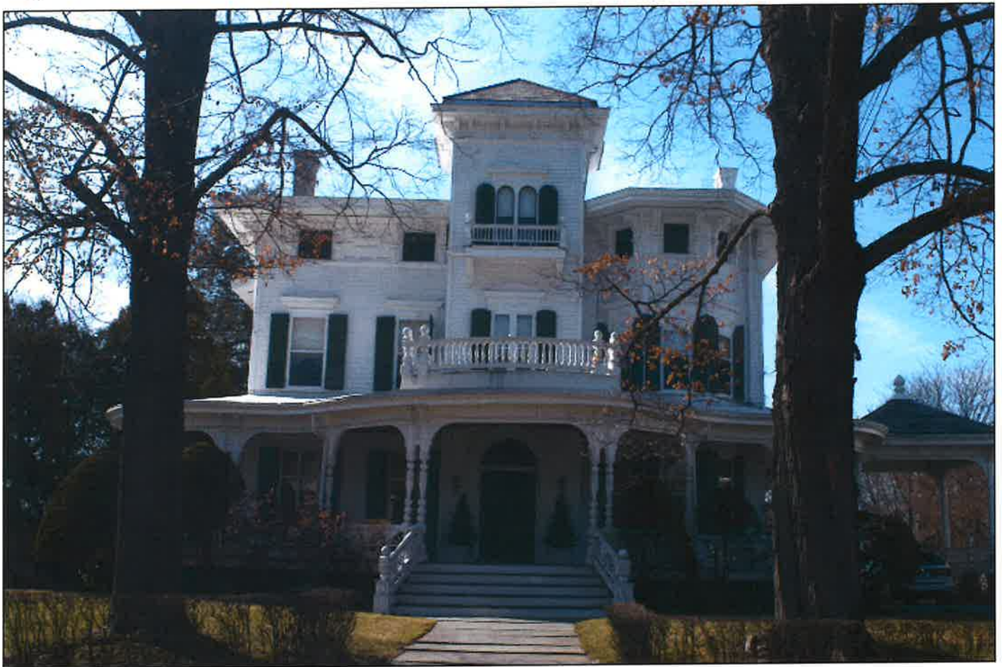
East (front) facade
