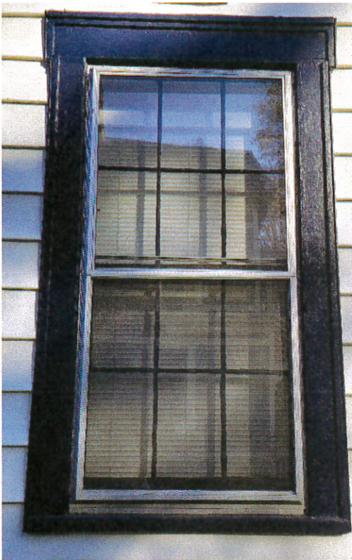
Existing window with Aluminum storm
