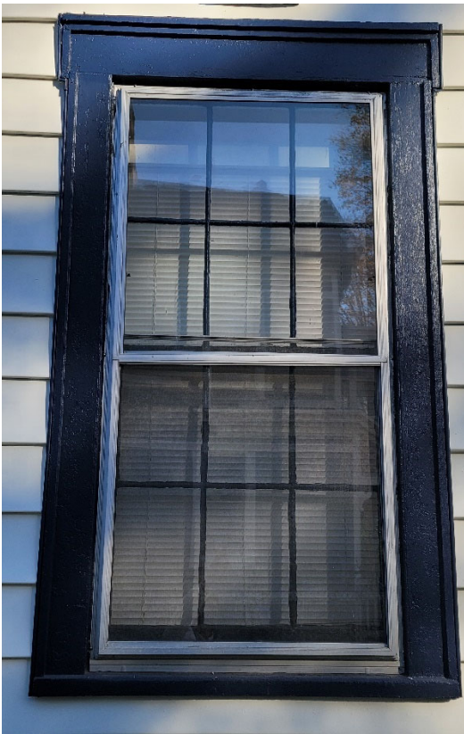
Existing window with Aluminum storm
