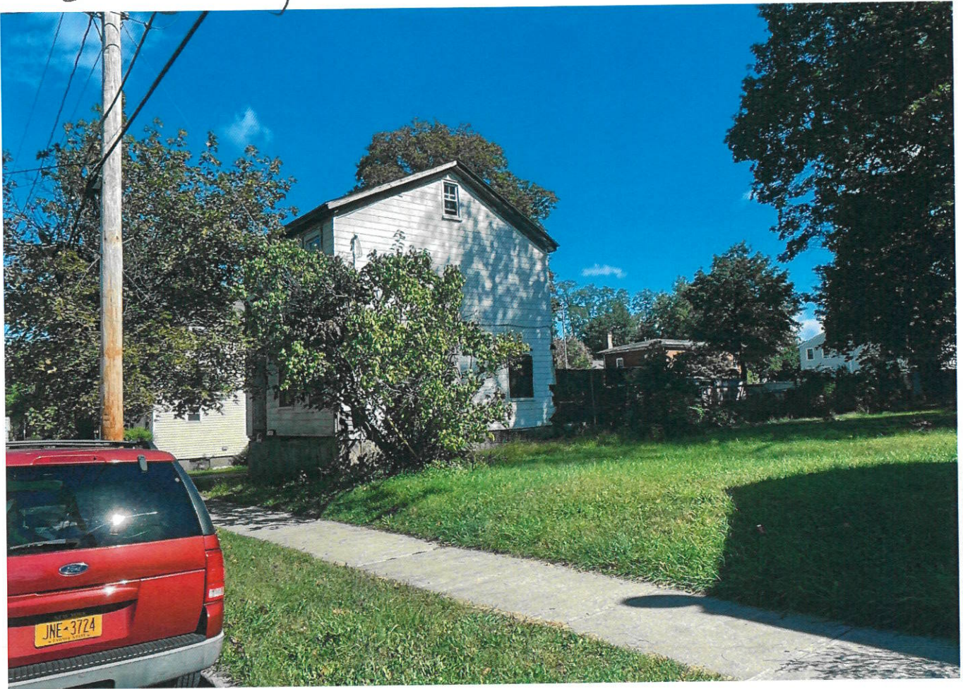
39 Pershing Ave. - Side View
