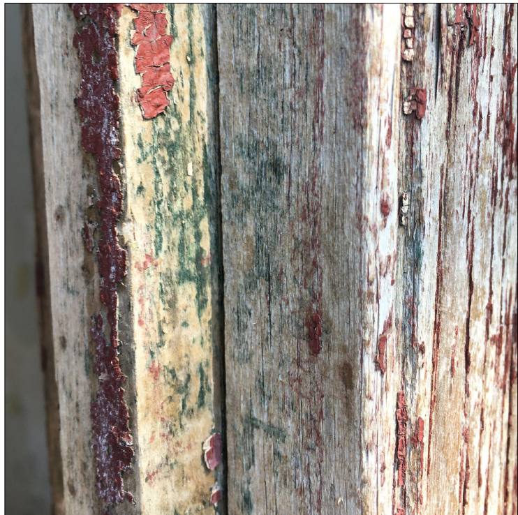
Evidence of a historic dark green window sash & brick mould paint finish was found at the remnants of front and rear windows where later dark red paint has flaked away or where gaps in trim have spread apart.
