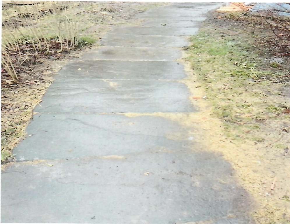
Existing frontyard bluestone walkway (existing bluestone re-set in stonedust)
