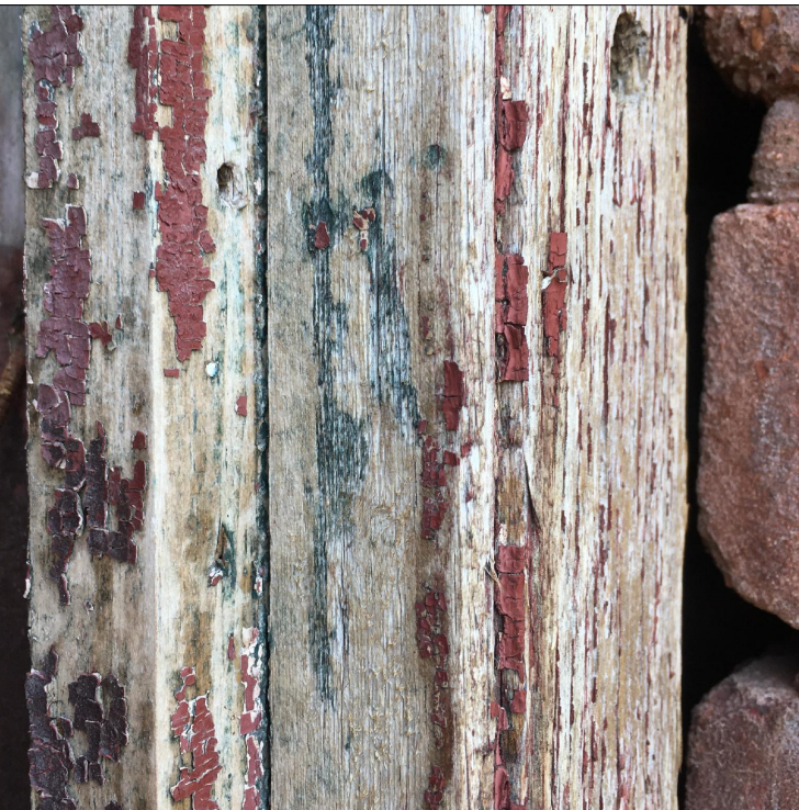
Evidence of a historic dark green window sash & brick mould paint finish was found at the remnants of front and rear windows where later dark red paint has flaked away or where gaps in trim have spread apart.
