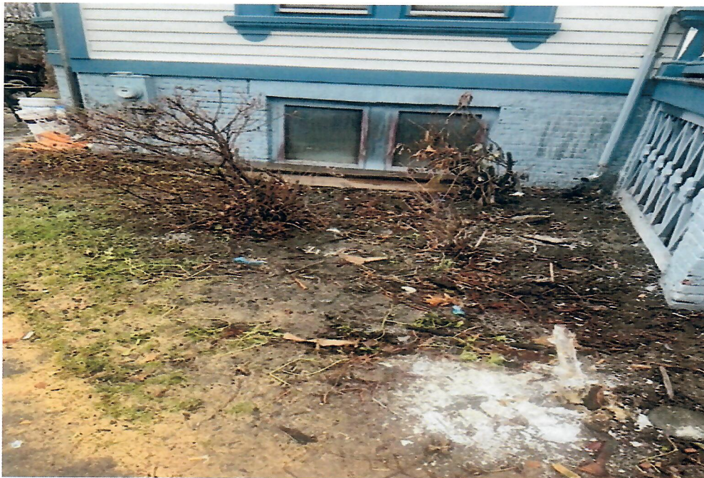
Existing left front yard next to house
