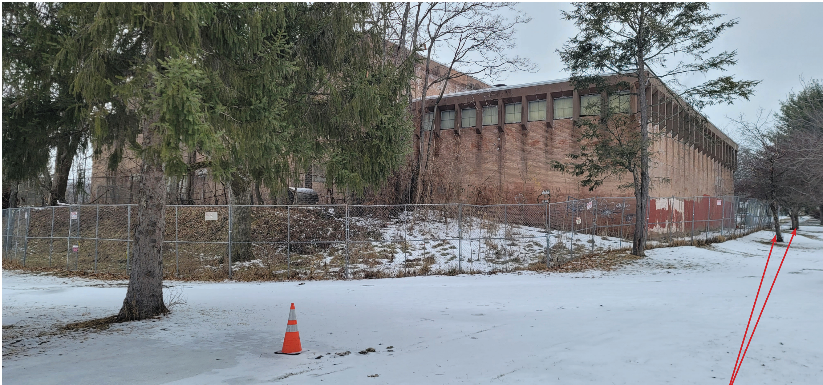
TREES ALONG PATH TO BE PROTECTED DURING DEMOLITION AND RECONSTRUCTION PROJECT
