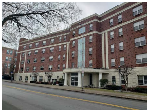
Rehab Adjacent to South
