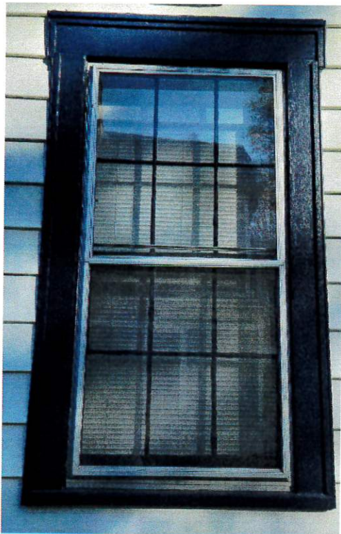
Existing window with Aluminum storm
