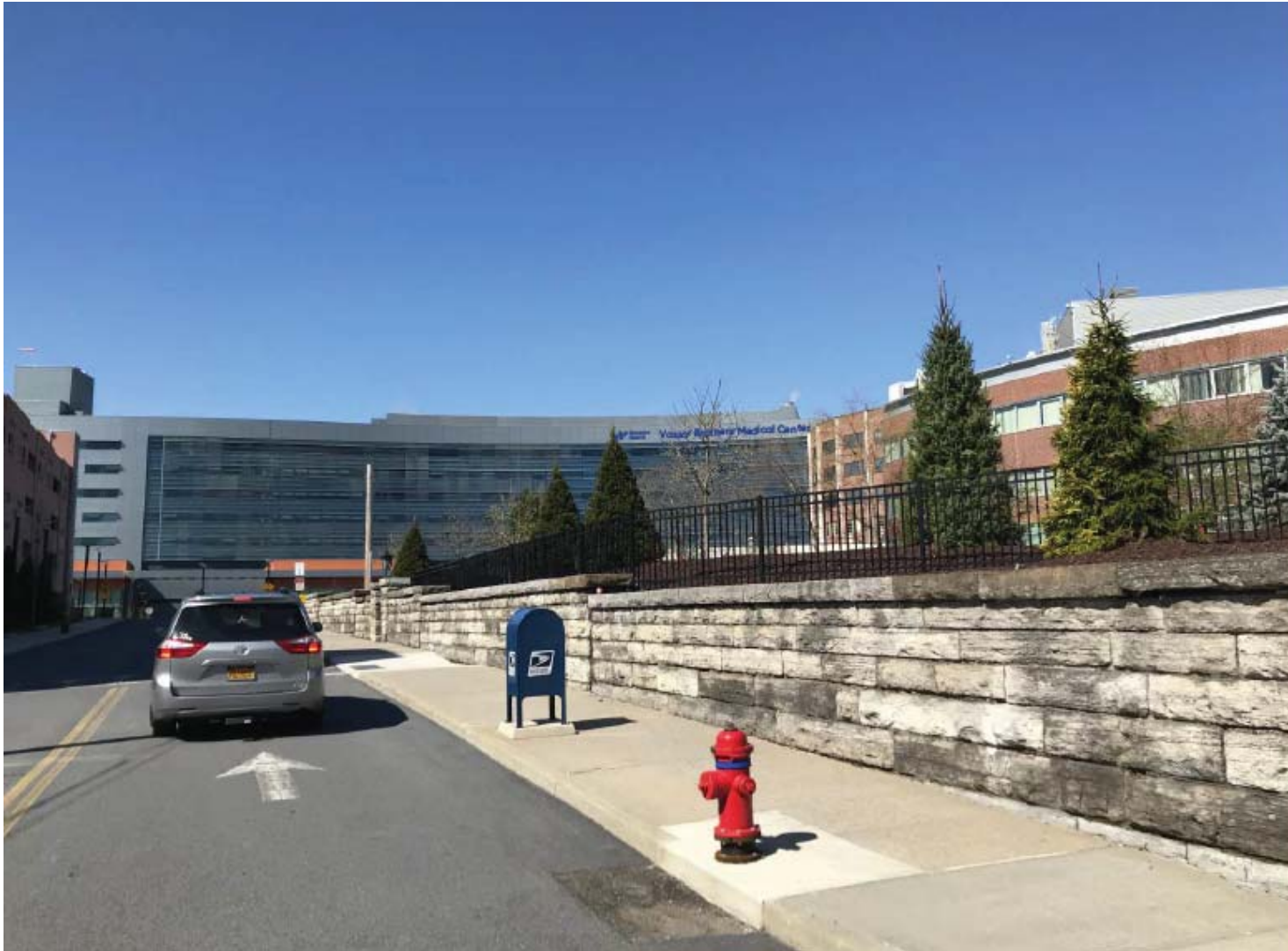
APPROACHING BUILDING ON LIVINGSTON FROM ±645' AWAY
