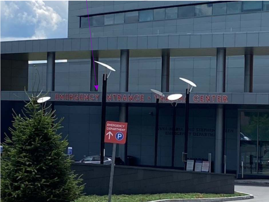
EMERGENCY DEPT. ENTRANCE - CLOSEUP
