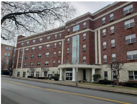
Rehab Adjacent to South
