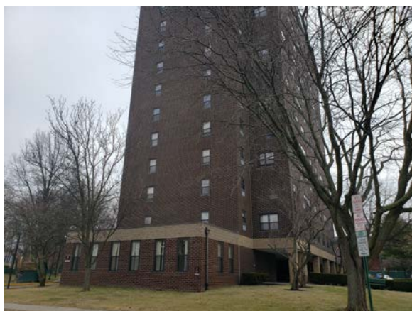
West Elevation of Property
