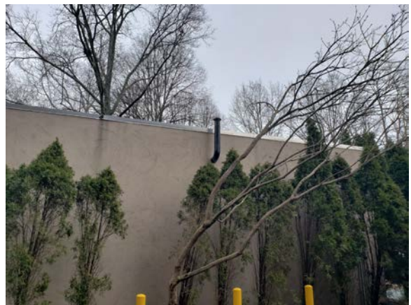
Vent Pipe on South Side of Tank House
