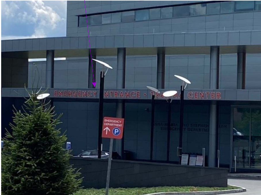
EMERGENCY DEPT. ENTRANCE - CLOSEUP
