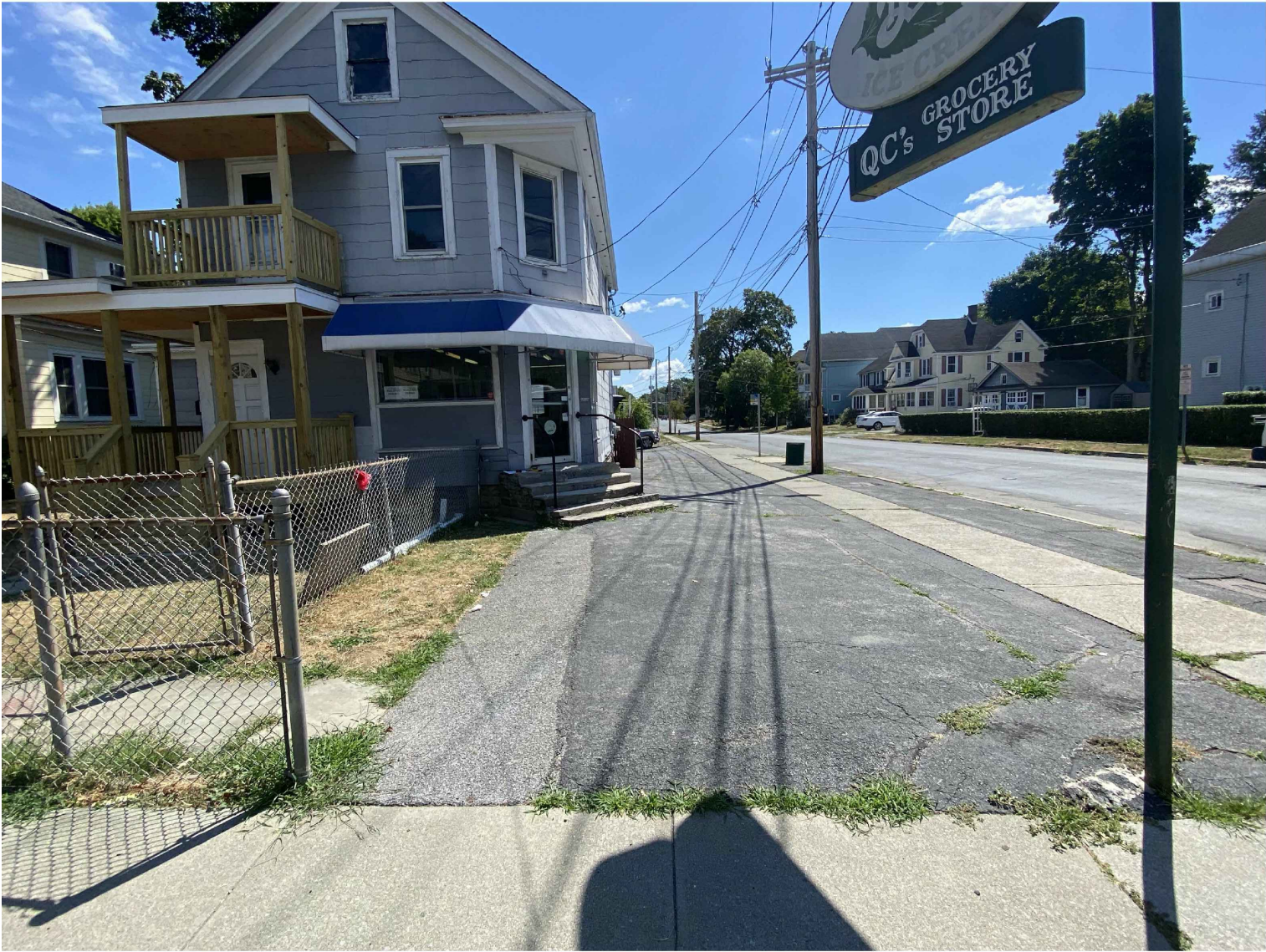
3 67 WORRALL AVE (looking east)
