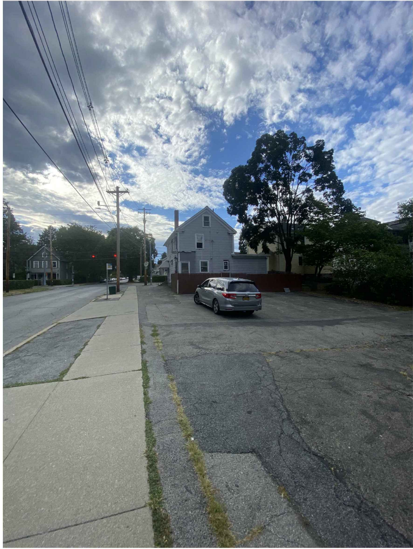
4 67 WORRALL AVE (rear yard / looking west)
