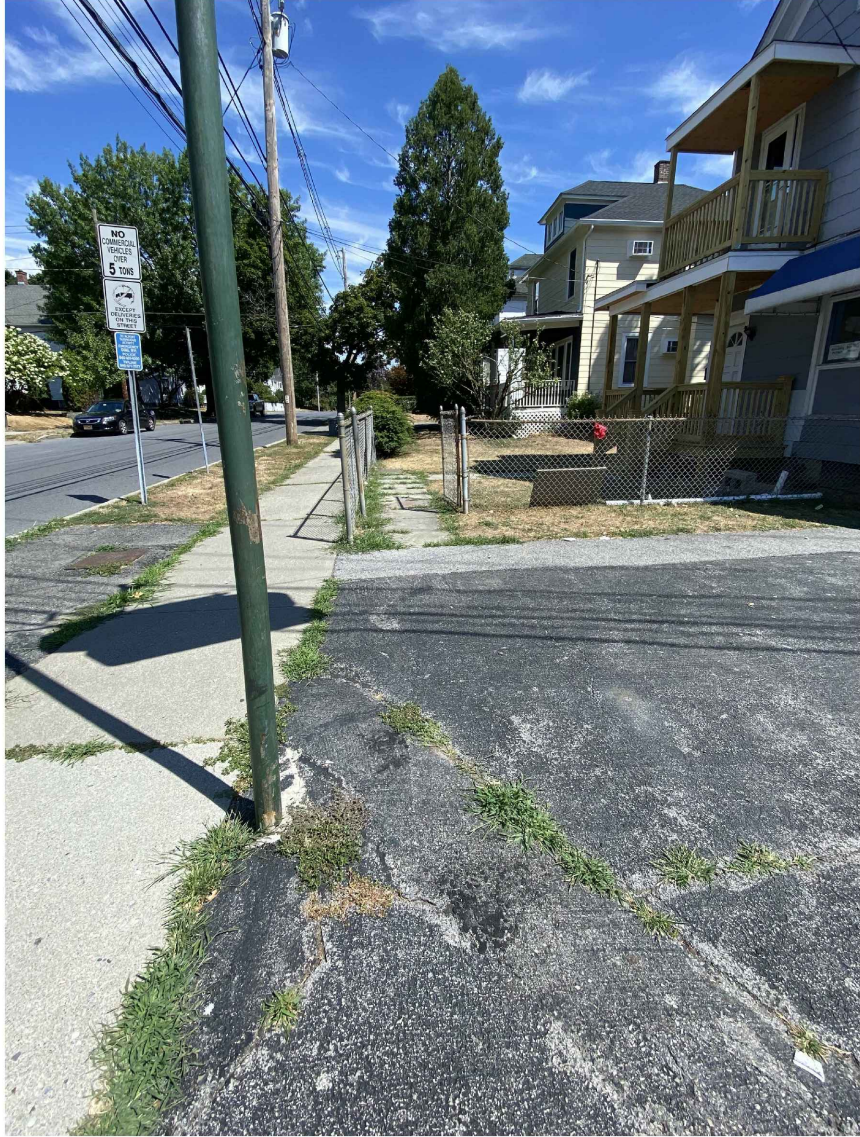
2 67 WORRALL AVE (looking north)
